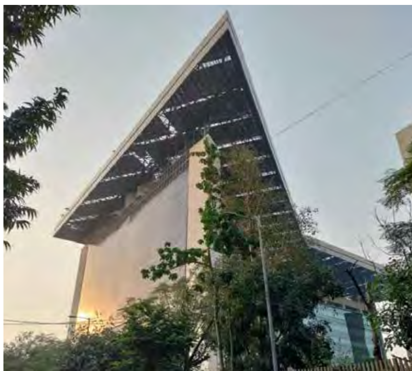
South-facing vertical façade of Atal Akshay Urja Bhawan featuring integrated solar panels
