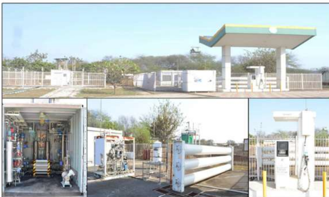
Fig.7.9: Centre of Excellence on Hydrogen Energy - India's first Solar based Green Hydrogen production cum dispensing station at NISE
