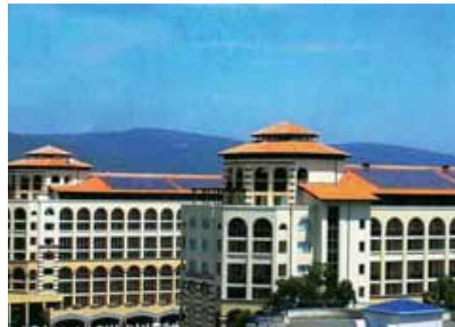
System integrated with building in a Hotel Source MNRE
