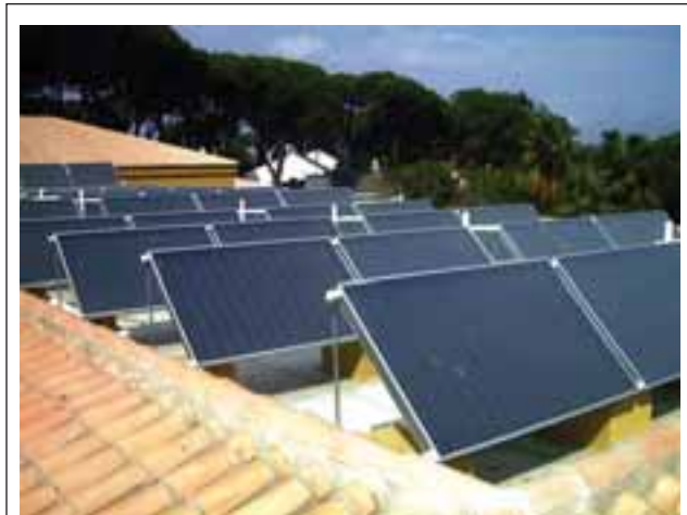
Figure 3 Flat plate solar collector panels installed in residential rooftops in Hawaii
