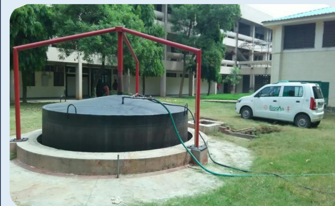
Car running on compressed biogas at IIT Delhi
