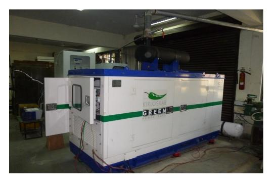
Figure 14: A photographic view of a hydrogen-fuelled generator developed in IIT Delhi with MNRE funds/support.
