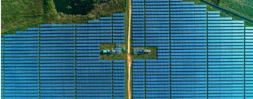
Figure 7-1: Utility scale PV plant
