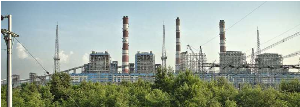
Figure 2-5: NTPC Barh Super Thermal Power Station (Ref. 17)
