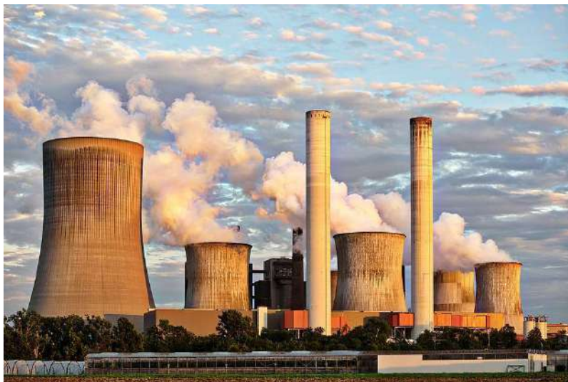
Figure 2-4: Vindhanchal Thermal Power Station, Madhya Pradesh (Ref. 16)
