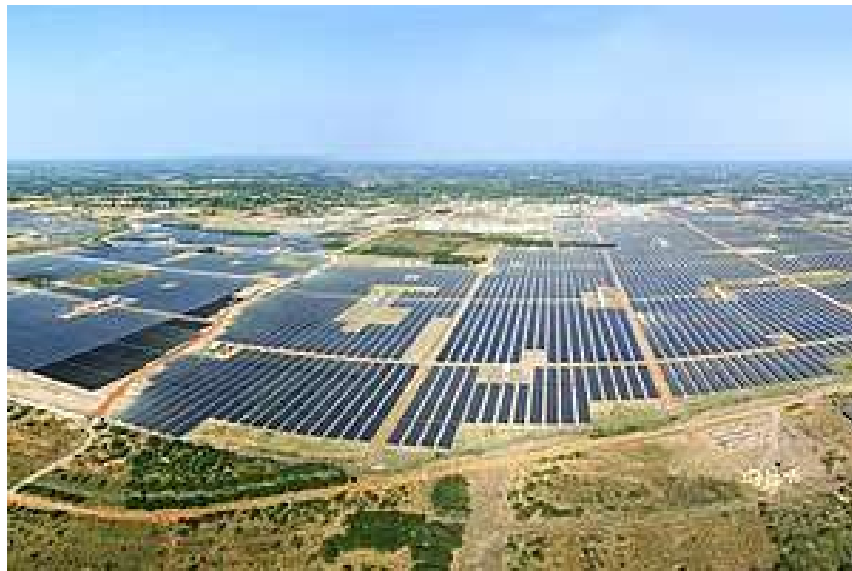
Figure 7-8: Kamuthi Solar Power Project (Ref. 11)
