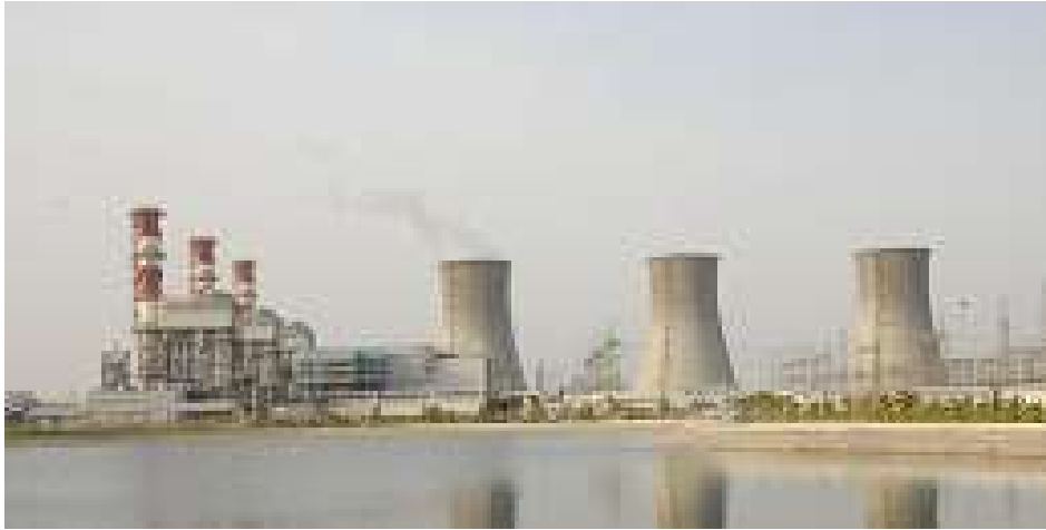
Figure 3-4 : Sugden Combined Cycle Gas Power Plant (Ref 14)
