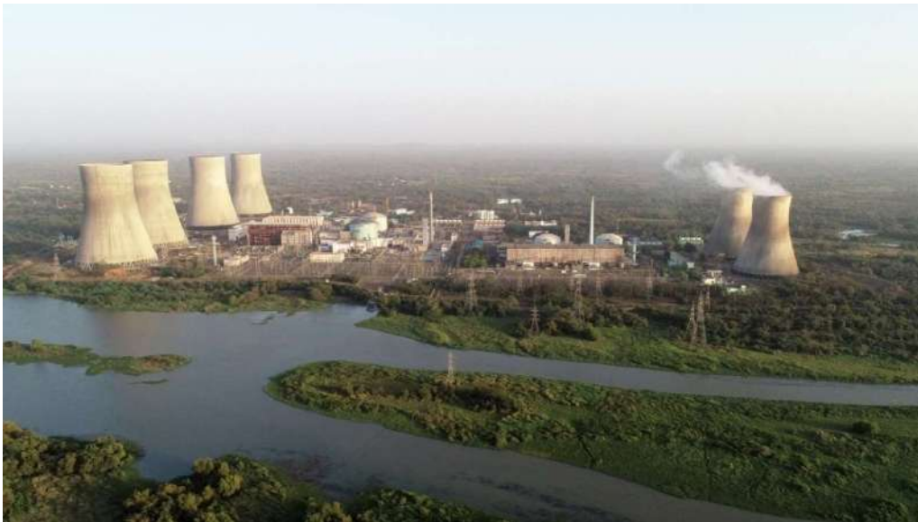
Figure 9-5: Kakrapar Atomic Power Station (Ref. 22)
