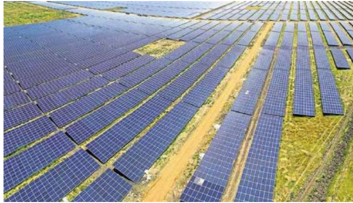
Figure 7-7: Rewa Solar Power Plant (Ref. 10)
