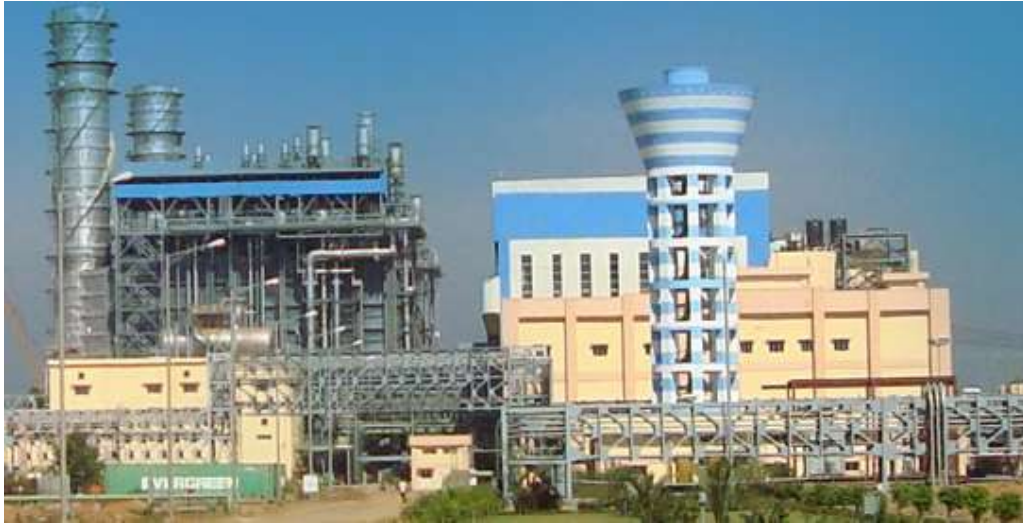
Figure 3-5: Tripura Combined Cycle Gas Power Plant (ref 19)
