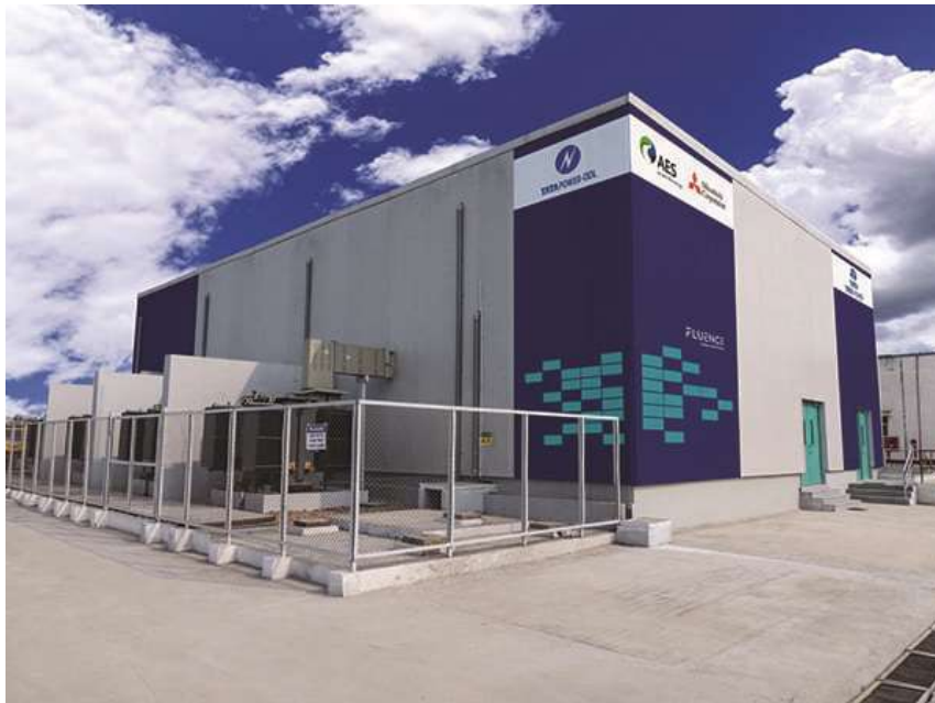
Figure 10-8: Rohini BESS, New Delhi (Ref. 46)
