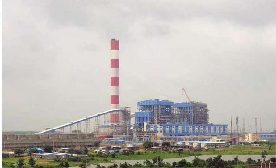
Figure 2-7: Khargone Power Plant (Ref. 19)
