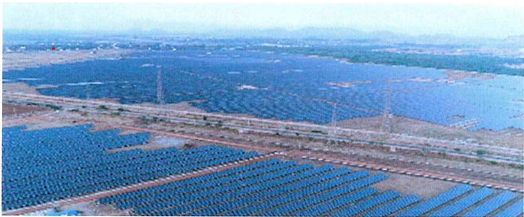
Fig. 1.2: Aerial view of Pavagada Solar Park
