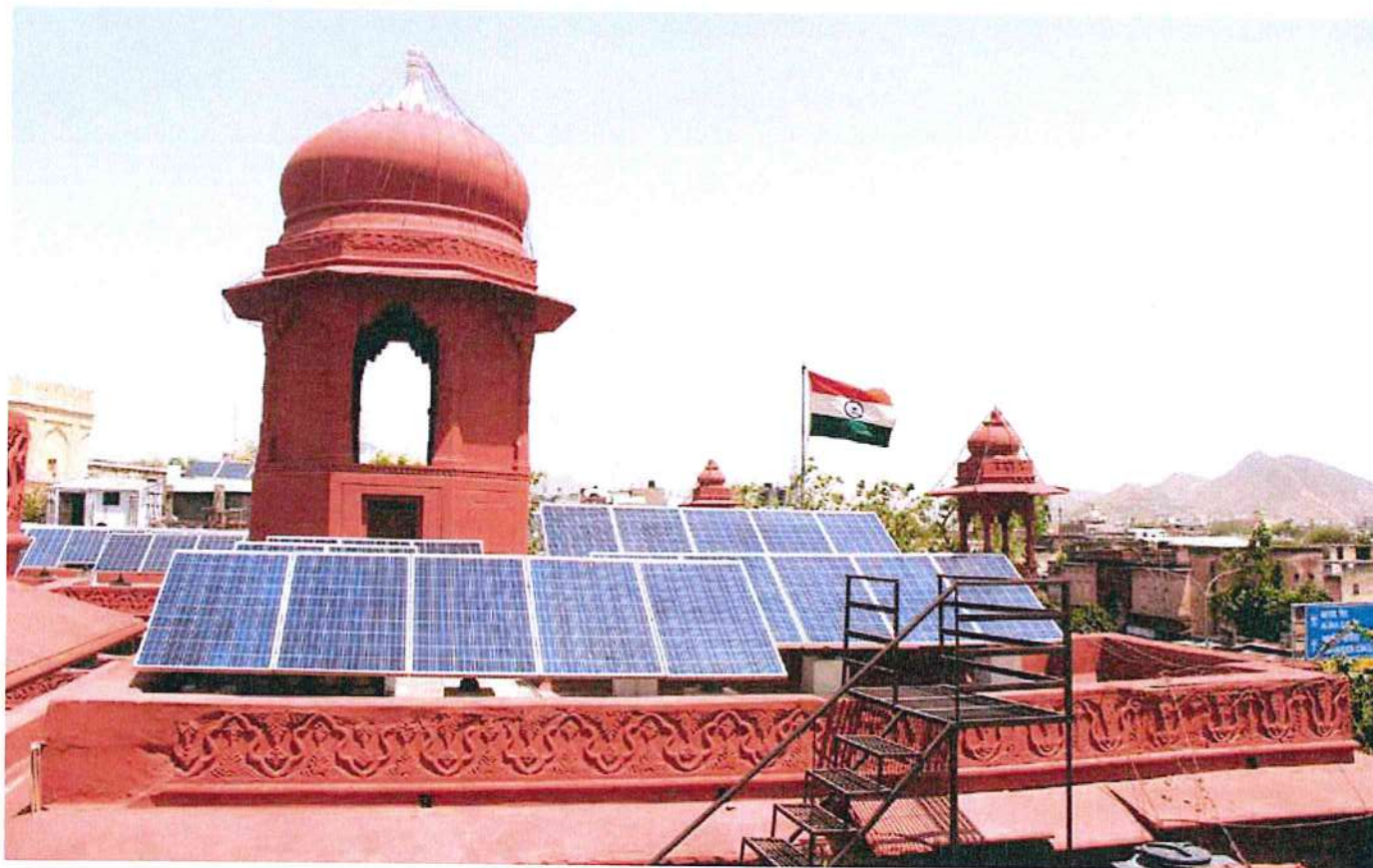
30 kWp Rooftop Solar PV Power Plant at Nagar Nigam, Ajmer, Rajasthan
