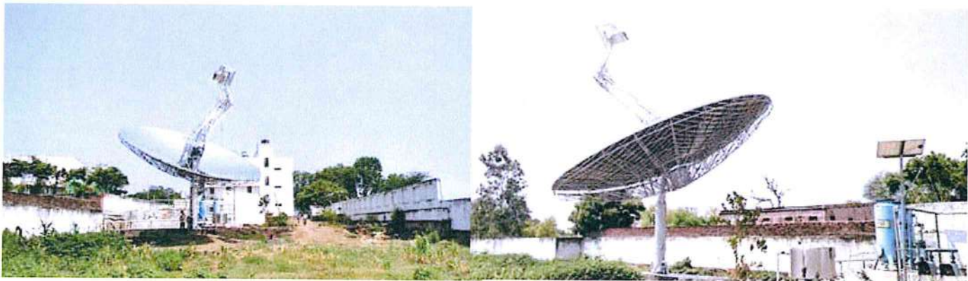
CST Installation at NIF, Kanpur, U. P.
