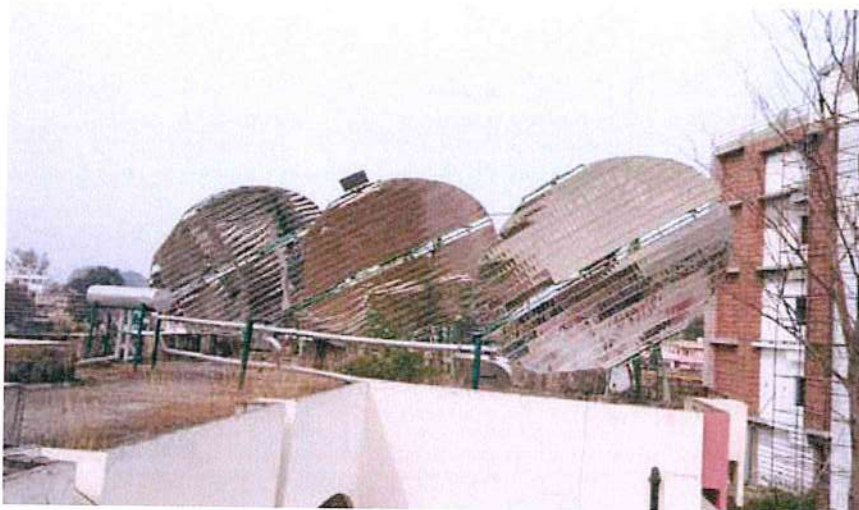
CST Installation at Youth and Sports Hostel, Una, Himachal Pradesh
