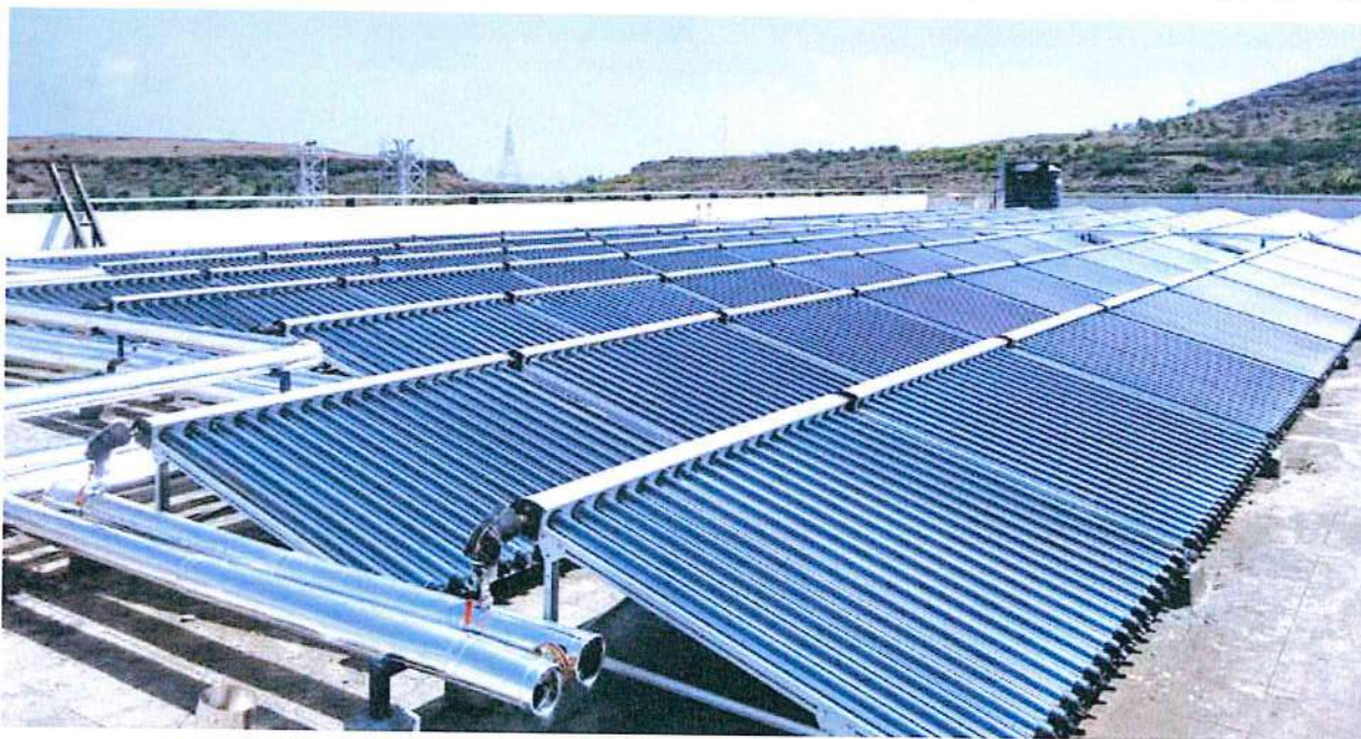
CPC based pressurized hot water system installed at Asian Paints Ltd., Khandala, Maharashtra
