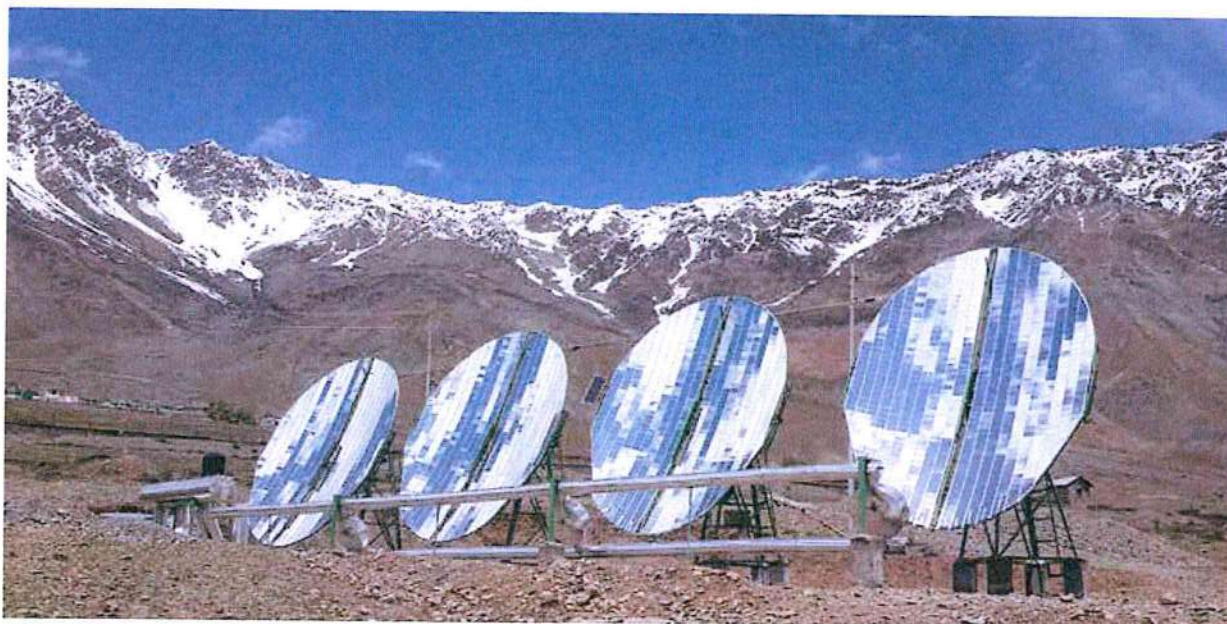
CST installation at Jawahar Navodaya Vidyalaya Campus, Khumbathang, Kargil
