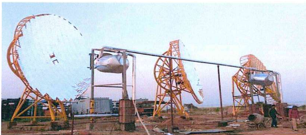
Fig. 7.8: Installation of Cast Iron receiver with piping and Insulation
