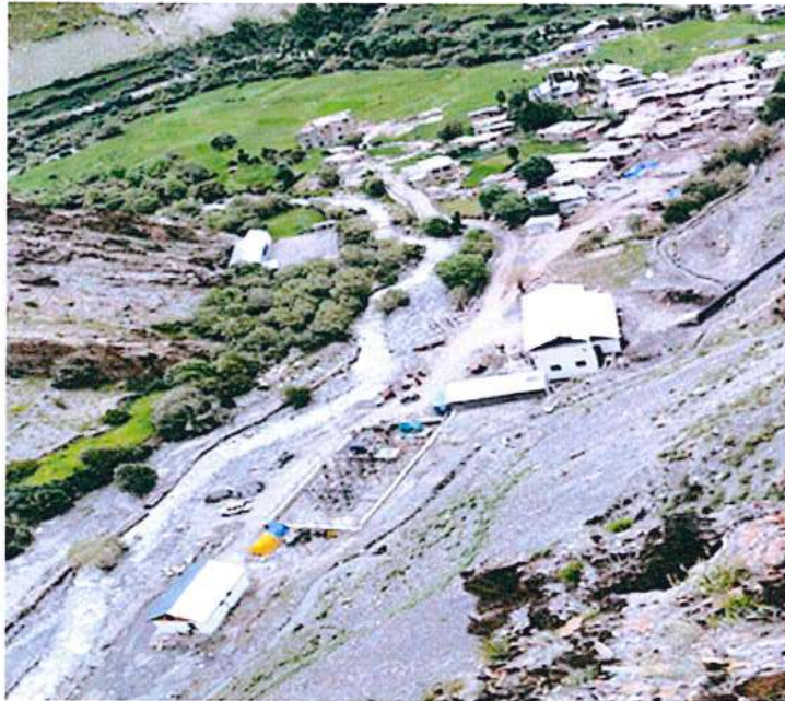
Fig.4.5: Khandi SHP (1000kW), District Kargil , UT of Ladakh – View of Power House & Switchyard
