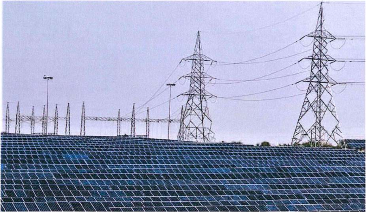
250 MW solar project in Rajasthan commissioned in FY 2019-20 (I)
