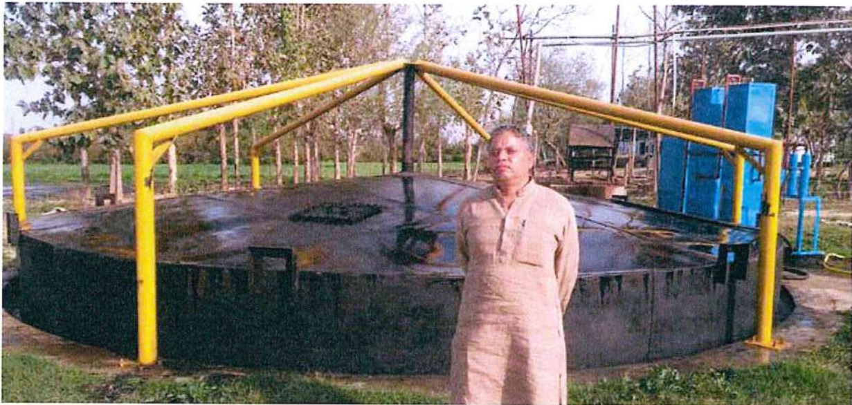
Biogas Power Generation (Off-grid) Project at site of beneficiary Sri Ramji Gupta, Vill- Bhatauli, Post- Rura, Dist- Kanpur Dihat (Biogas Capacity 140 m 3 / 16 KW)
