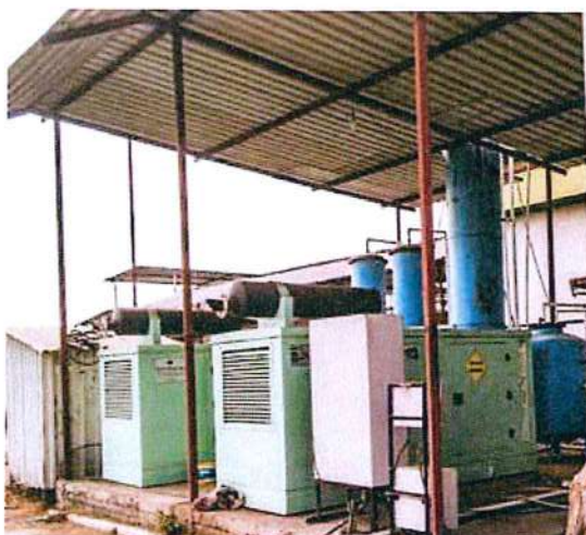
Biogas plant of 650 m 3 / 75 kW Biogas Power (Off-Grid) project at M/s. Bhagya Laxmi Dairy Farm, Village Sultanpur, Post-Manchar, Taluka- Ambegaon, District - Pune (Maharashtra)
