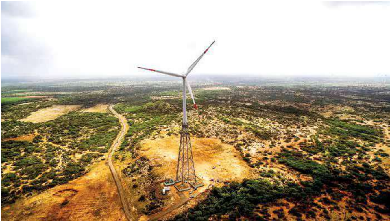
Wind Turbine with Hybrid Lattice Tower installed in Kutch, Gujarat
