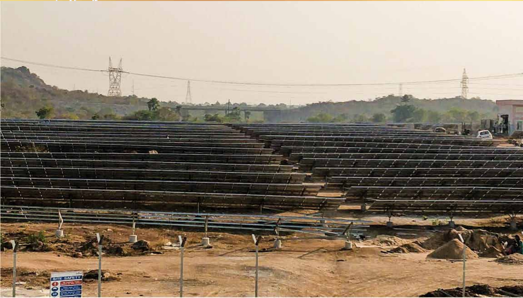
5 MW solar project at BDL, Ibrahimpatnam (under construction)
