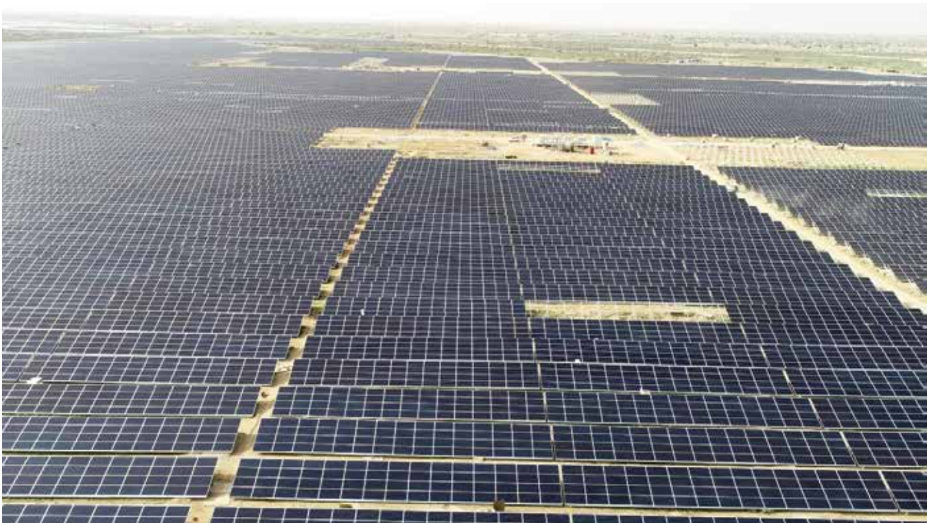
10 MW solar project in Rajasthan
