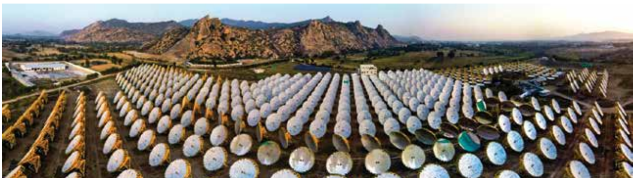
1 MWe (3.5 MWth) solar thermal power plant with 16 hours thermal storage (770 solar dishes) at Mount Abu, Rajasthan
