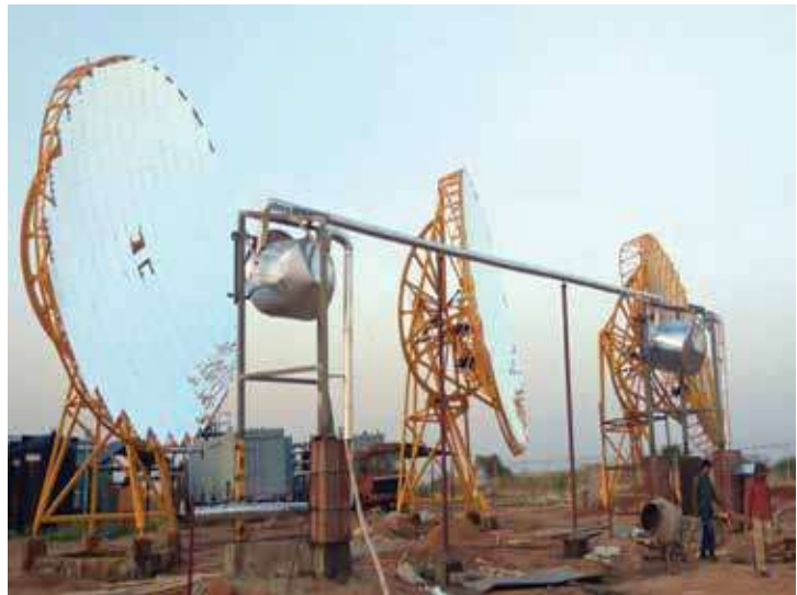
Installation of cast Iron receiver with piping and Insulation
