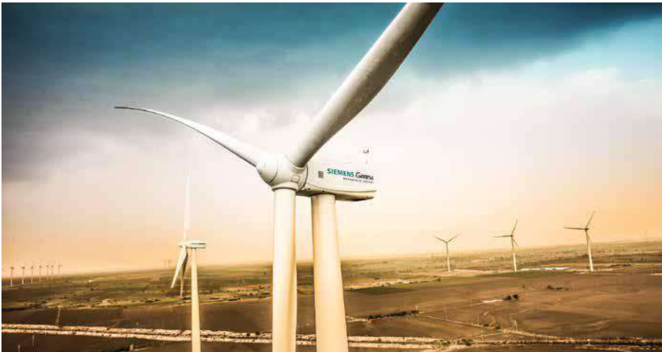
200 MW wind farm at Ananthapur, Andhra Pradesh
