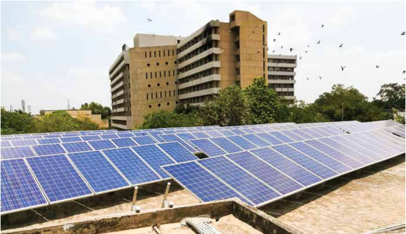
Geological Survey of India, Lucknow
