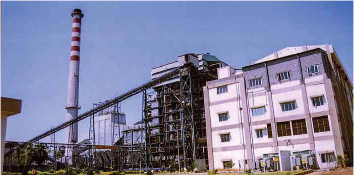
24 MW Bagasse Based Co-generation Power Plant, Kukkuwada, Tehsil & Dist. Davangere, Karnataka
