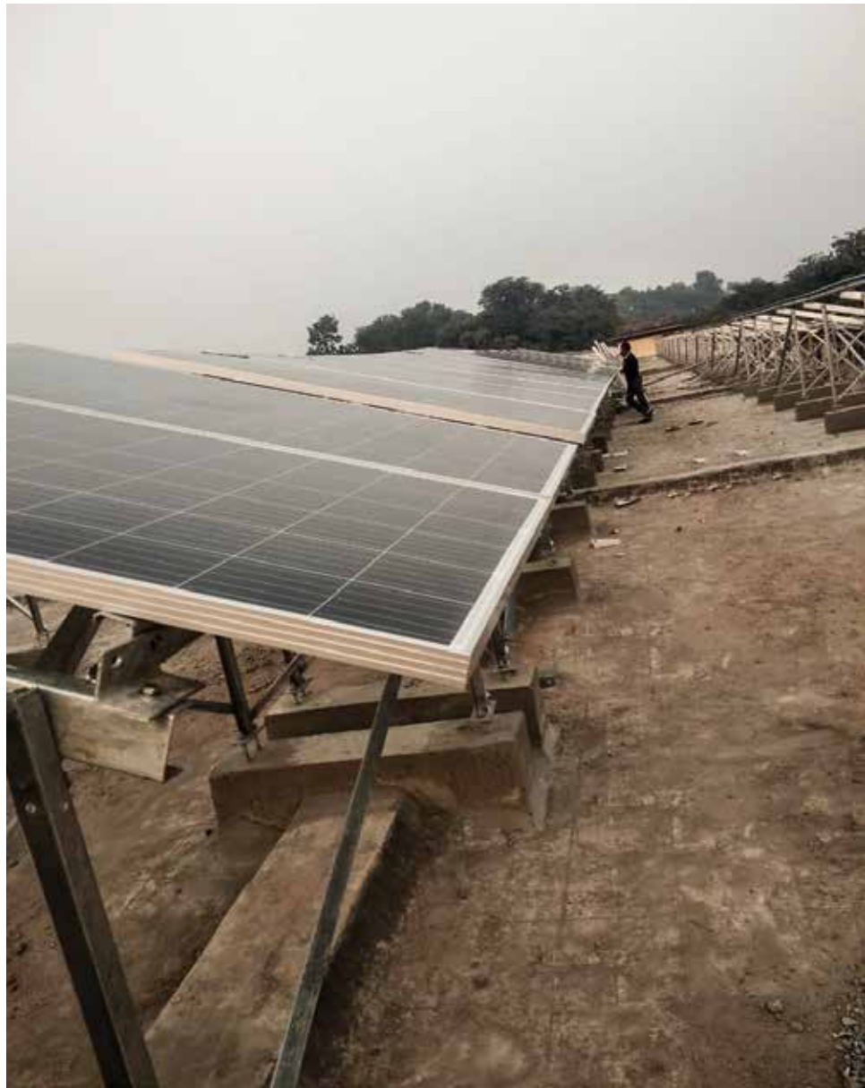
Rooftop solar project at BHU (under construction)
