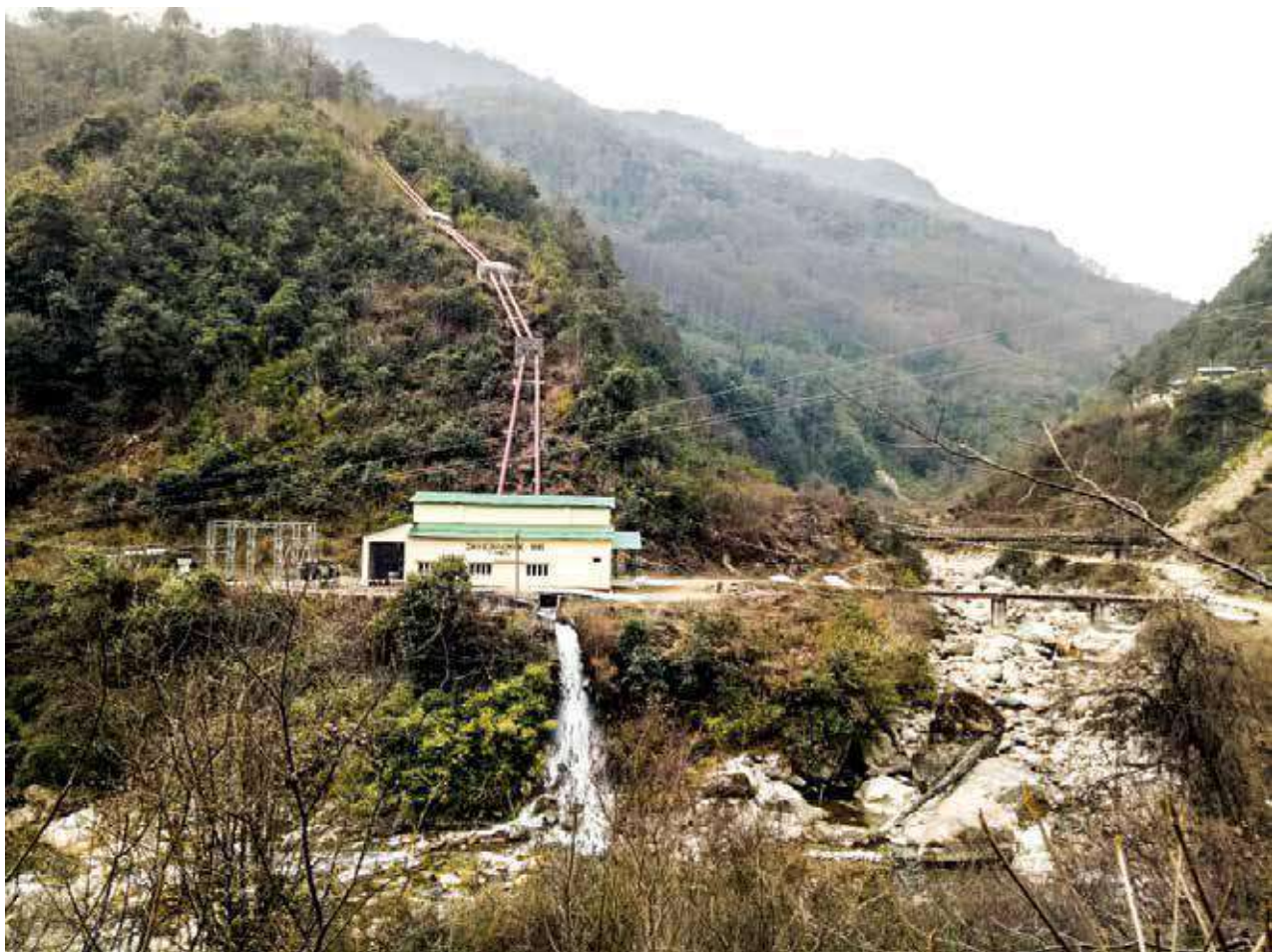
The 1 MW Zhangdongrong SHP in West Kameng District of Arunachal Pradesh under package for illumination/electrification of Villages located in Border Districts
