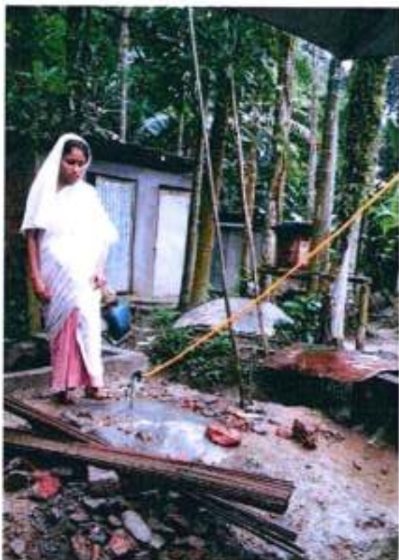
3 m 3 capacity Deenabandhu model biogas plant at Village Dholbari, P.O-Dholbari, Dist-Lakhimpur, Assam,
