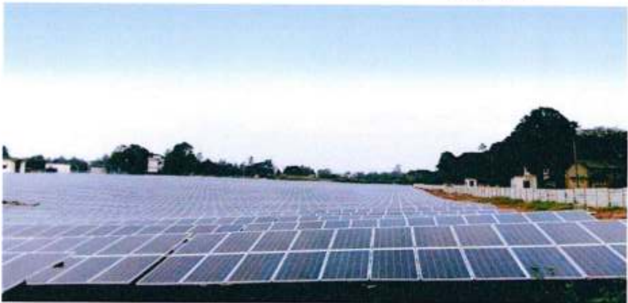
4 MW New Mangalore Port Project
