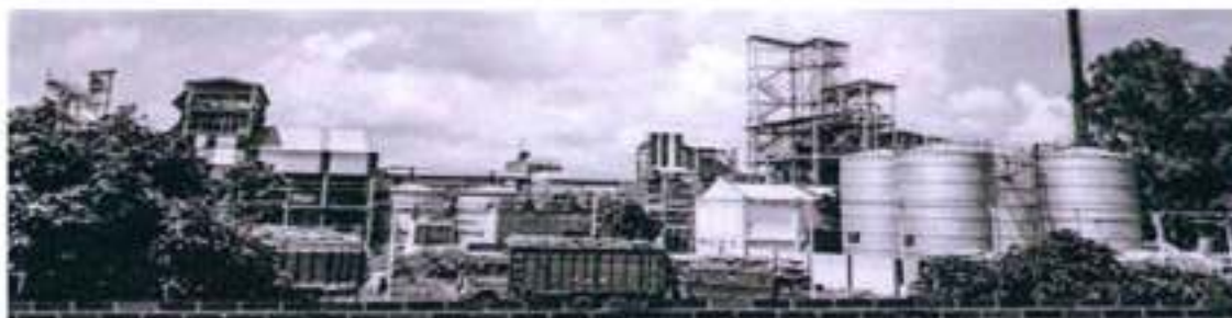
1.5 MW biomass co-generation project installed at Sansarpur Terrace, Kangra, Himachal Pradesh
