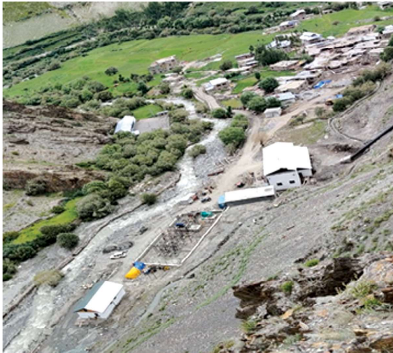
Fig.4.5: Khandi SHP (1000kW), District Kargil , UT of Ladakh – View of Power House & Switchyard
