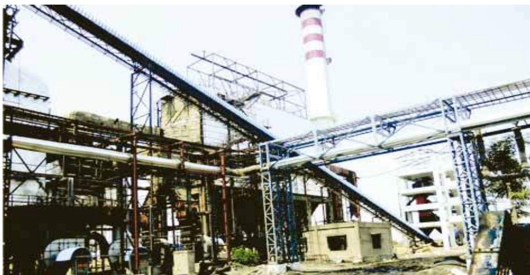
1.0 MW biomass co-generation project installed at Vill. Karambedu, Dist. Thiruvallur, T.N
