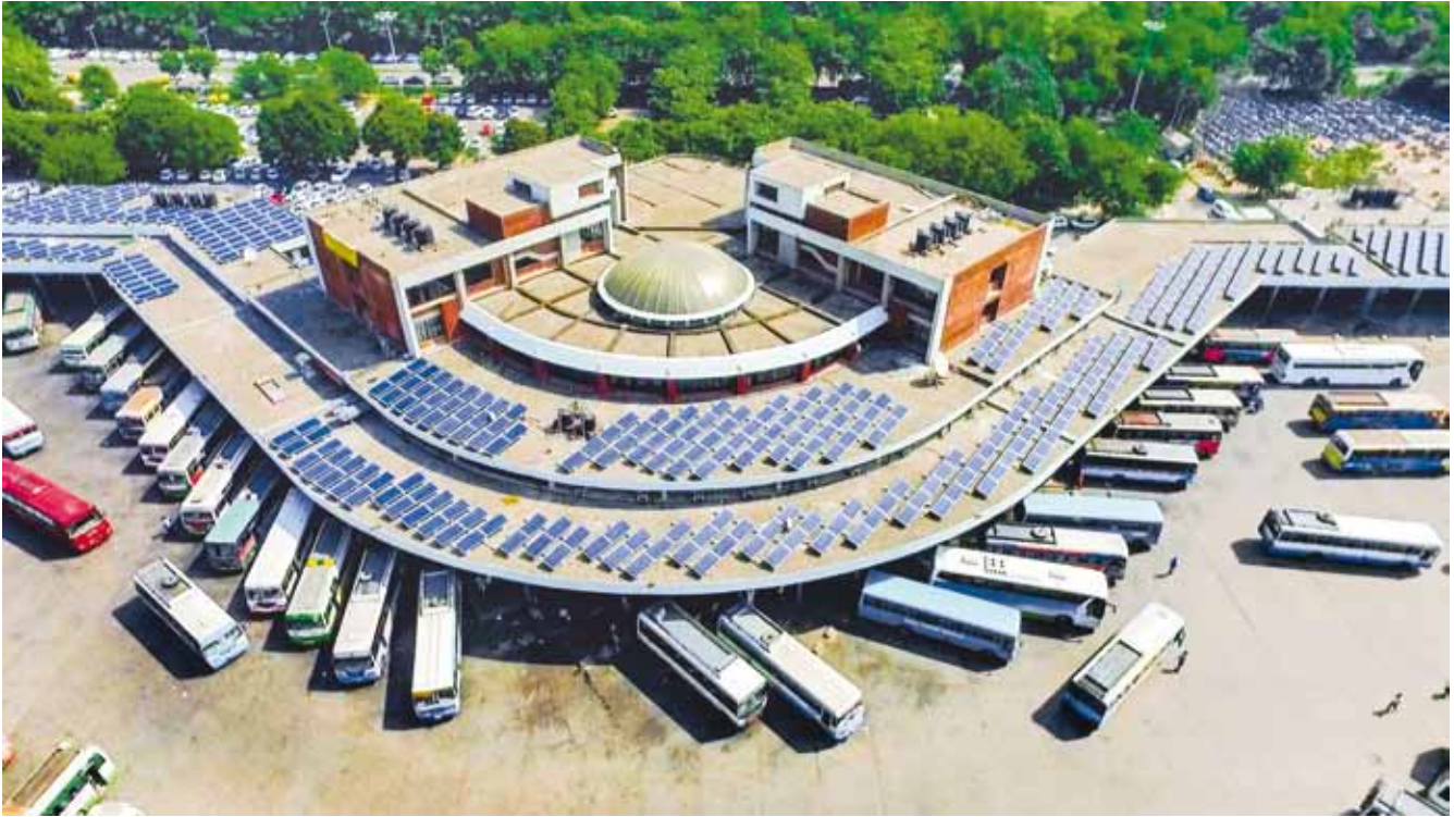
SPV Power Plant at ISBT Sector-43, Chandigarh under Model Solar Cities Programme
