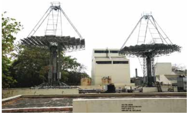
Installation of 338 sq. m of ARUN Dish at Aavin Dairy, Salem
