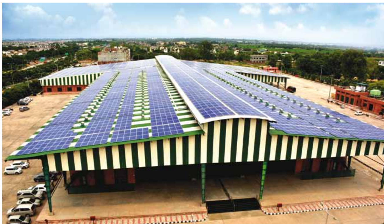
10MW Grid connected Solar Rooftop Power Plant, Punjab
