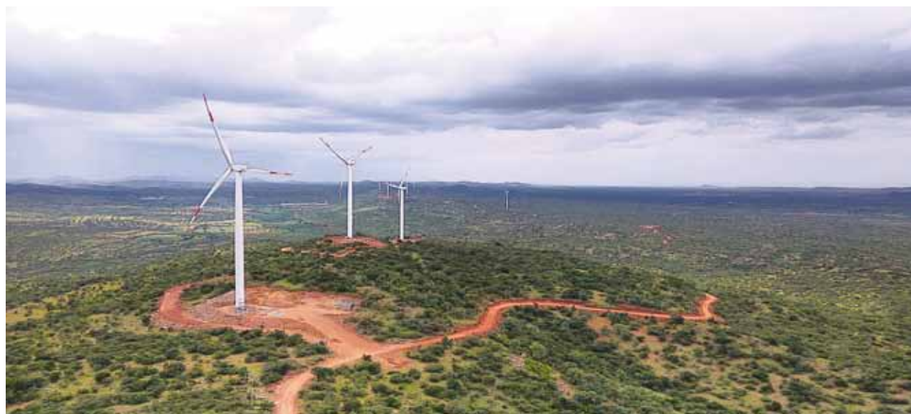
119.7 MW wind farm in Ellutla, Andhra Pradesh
