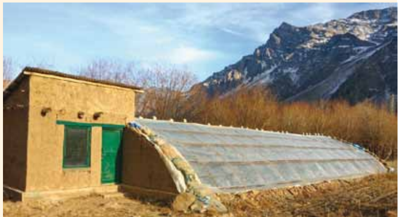
Installation of Domestic Type Green House in Kargil region
