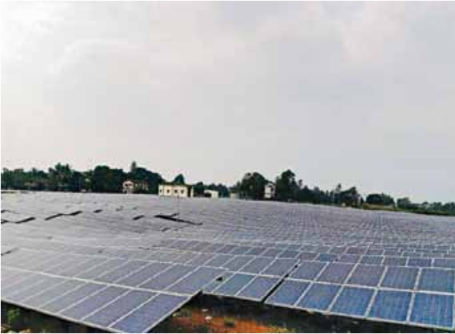
4 MW New Mangalore port under SECI PMC Works
