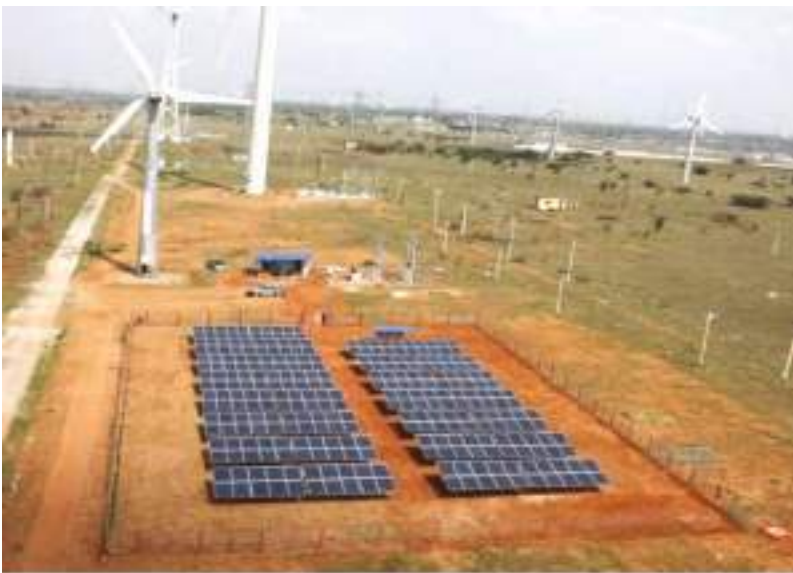
Grid integration of 75 kW solar with 200 kW WEG
