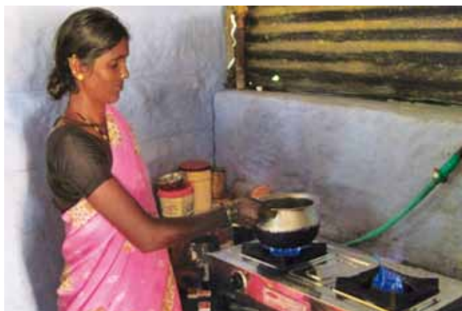
Biogas generation and use in kitchen by the beneficiary Smt. Chintha Vijaya Laxmi, W/o- Shri Chintha Laxmi Kantha Reddy, Vill. – Puttapasham, Mandal – Gonegandla, Dist. – Karnool (AP)
