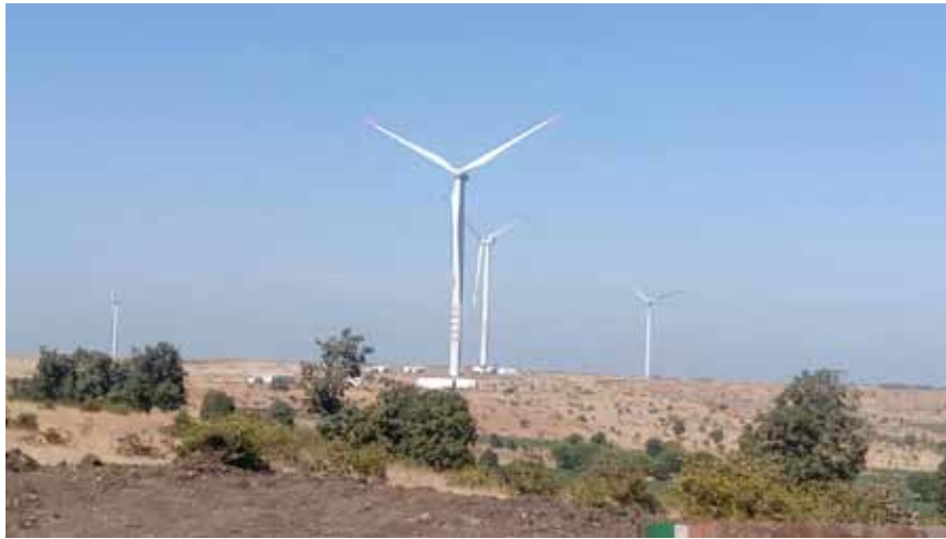
92 MW Lahori Project in Madhya Pradesh
