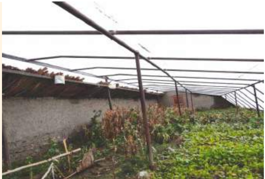
Inside view of Commercial type Green House installed in Kargil region
