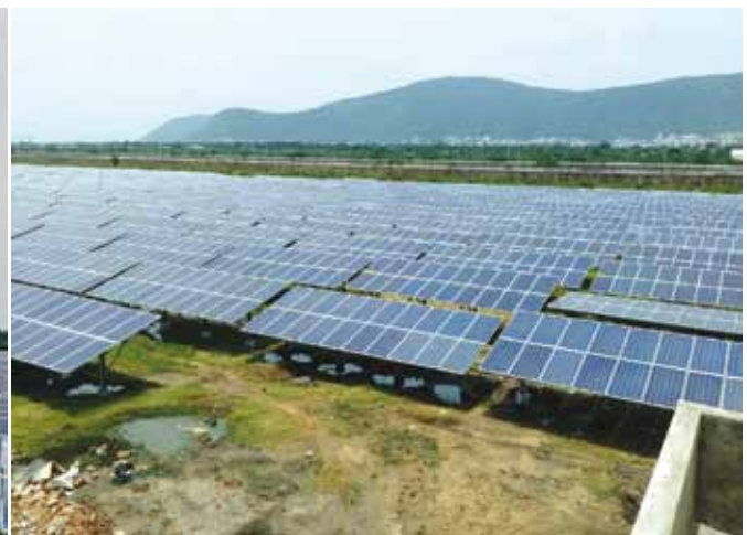
Project at Vishakhapatnam port under SECI PMC Works
