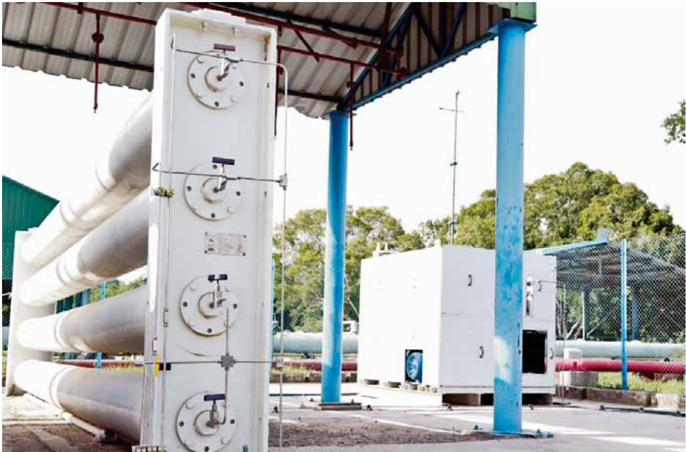
High Pressure storage tube (Left) and Compressor (Right) at IOCL R&D Centre Faridabad
