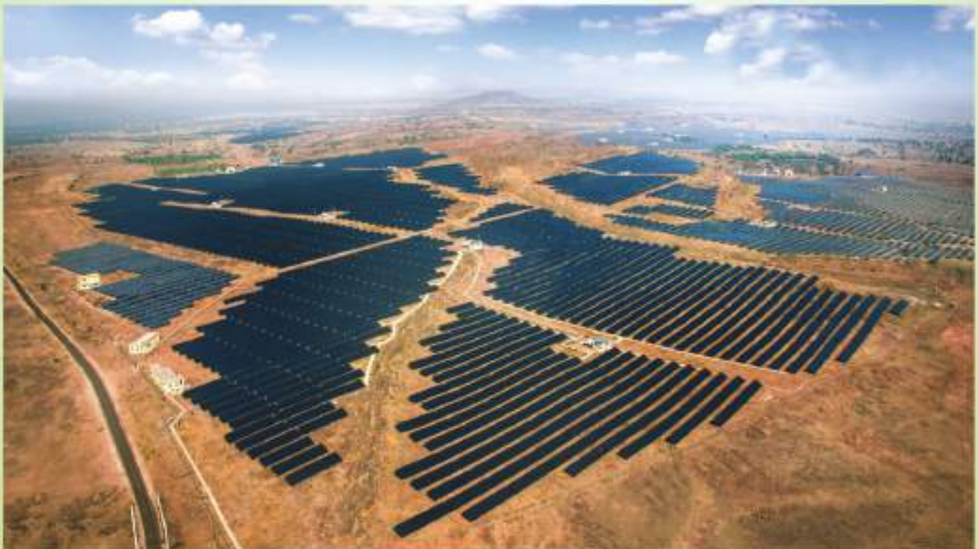
100 MW Solar PV Power Plant in Jodhpur
