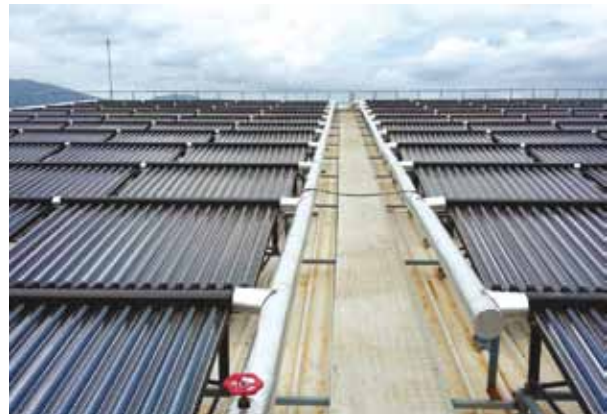
Installation of 721 sq. m NIC solar system at Hatsun Agro, Salem
