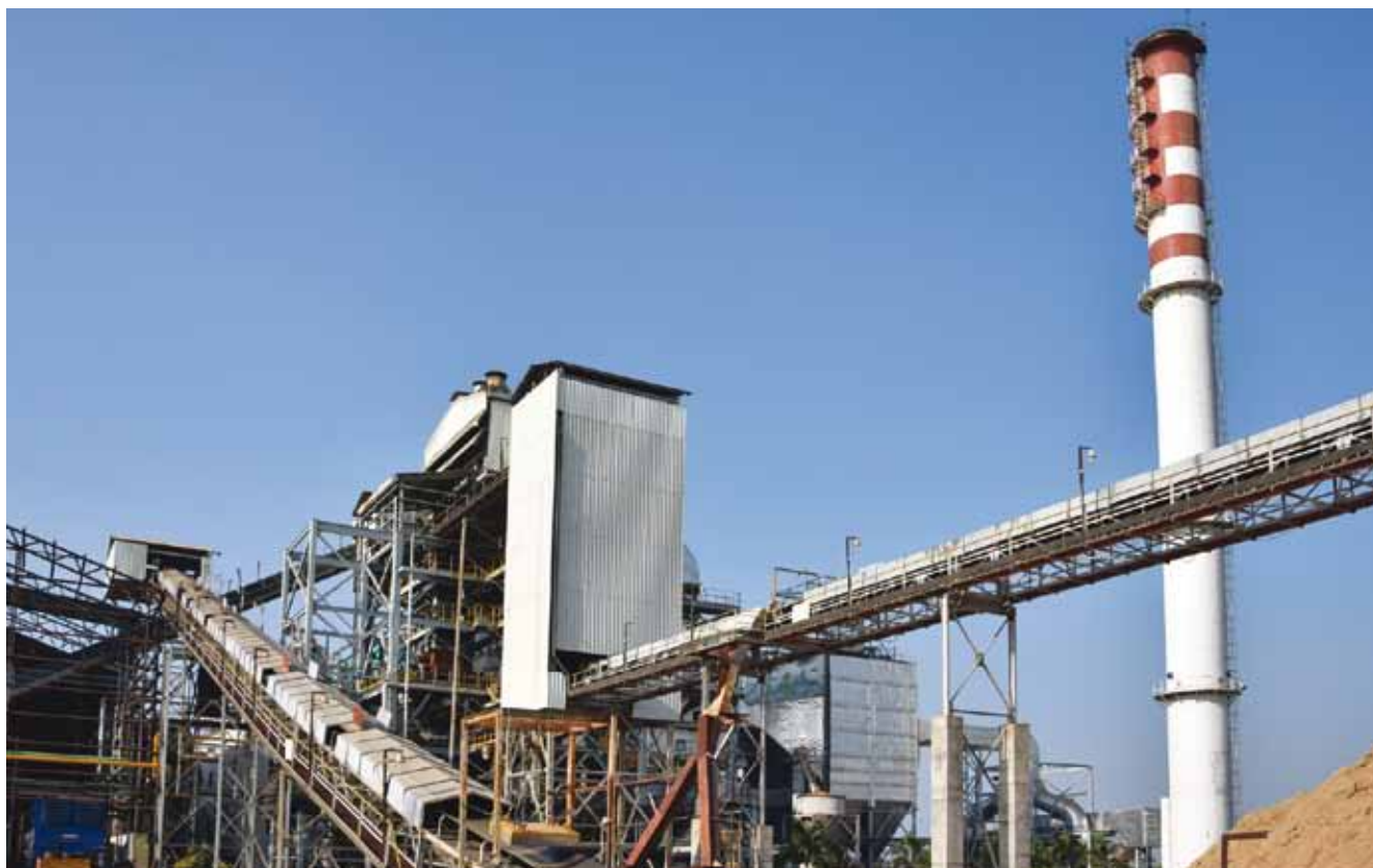
A 14.8 MW Cogeneration project at Saswad Mali Sugar factory Ltd, Malinagar, Dist. Solapur, Maharashtra
