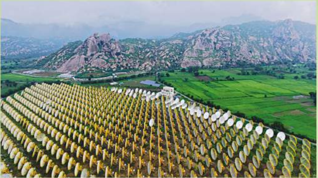
1.0 MW Solar Thermal Power Plant with 16 hr. Thermal Storage in Brahmkumari Ashram, Mount Abu
