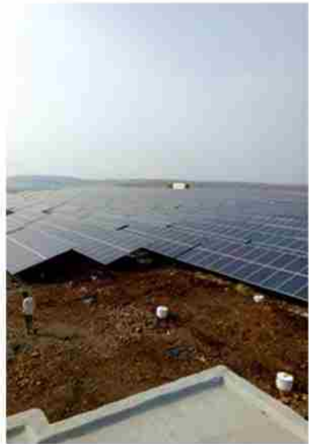
10 MW Solar Power Project in Maharashtra
