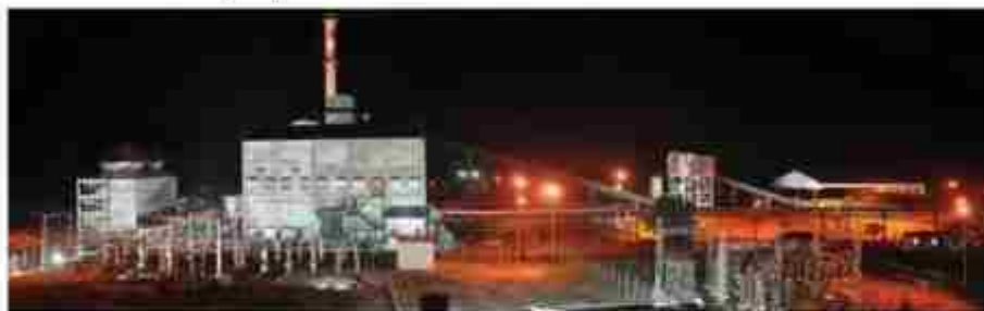
8 MW Biomass based Power Plant (Manas Agro Unit-2 / previously known as "Yash Agro") situated at Village - Kolari, Dist- Chandrapur, Maharashtra.
