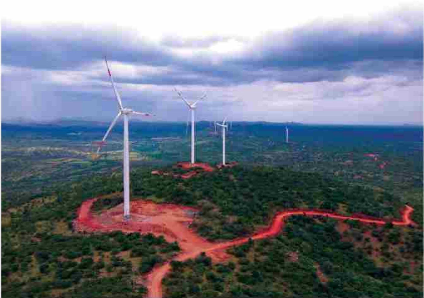
120MW wind farm at Anantpur in Andhra Pradesh
