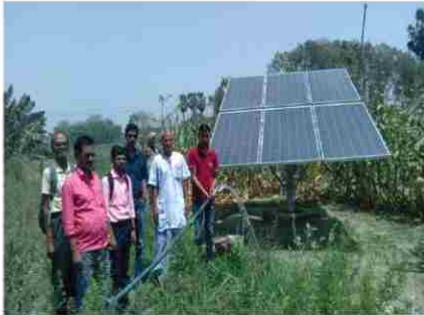
2 HP Solar Water Pumping Systems installation under irrigation scheme in Bihar
