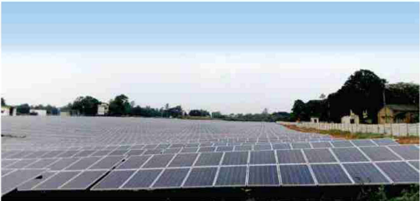
4 MW New Mangalore Port Project
