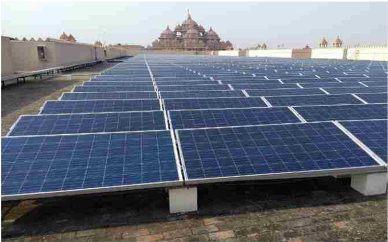
Grid connected solar rooftop plants of 650 kWp installed by SECI at BAPS Swaminarayan Sanstha, Pandav Nagar, New Delhi
