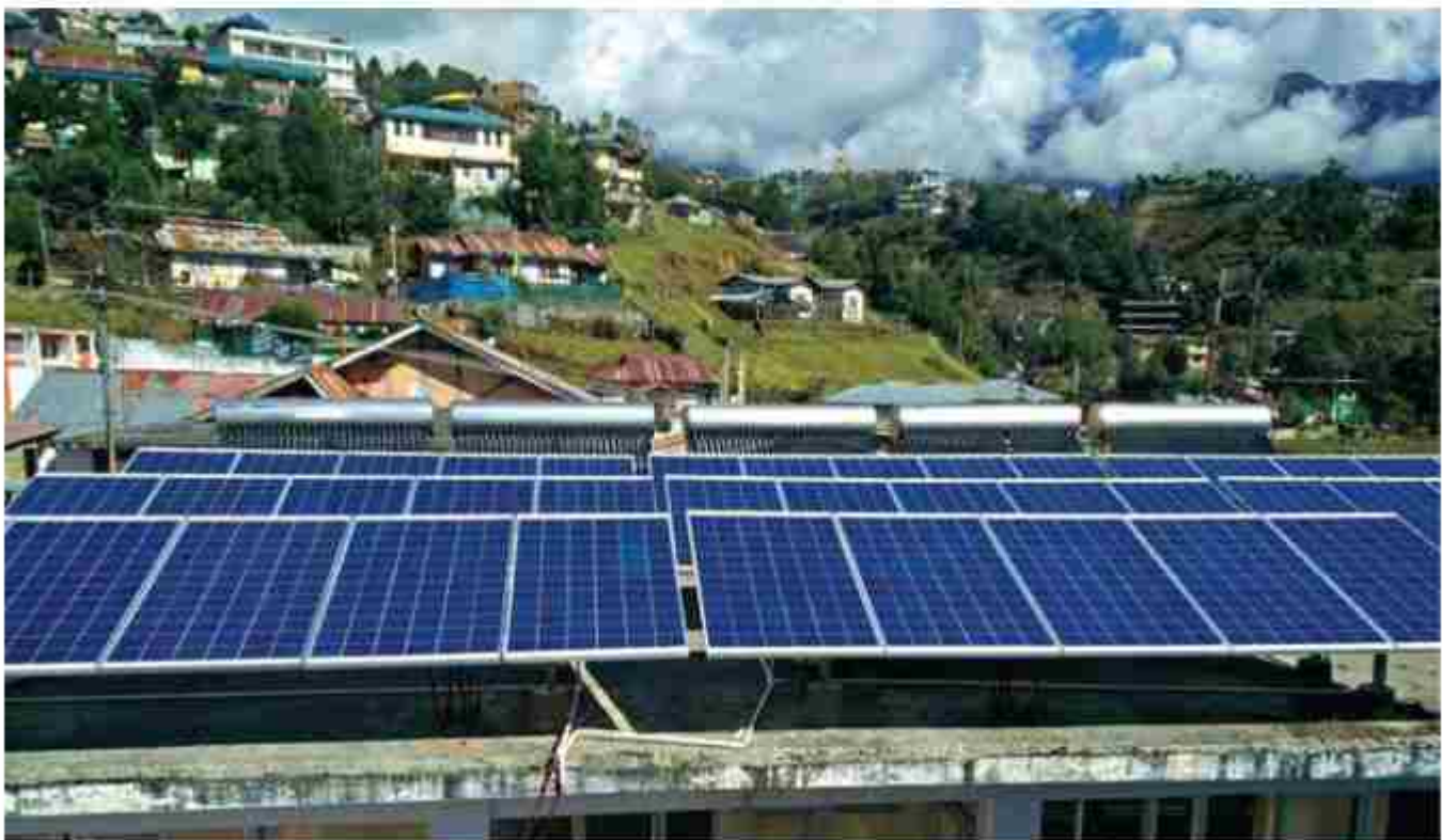
Solar Photovoltaic Power plant and Solar Water Heating Systems at District hospital in Arunachal Pradesh
