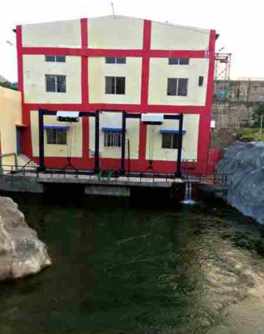
2x1.5 MW SHP project at North feeder canal of Somasila Reservoir in Andhra Pradesh
