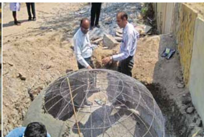
2m3 Deenbandhu ferro-cement Biogas Plant under construction at village – Guntappa, Mandal – Guduru, Dist. – Karnool (AP)
