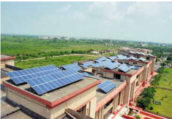
500 kW Solar Power Plant at High Court Bilaspur, Chhattisgarh
