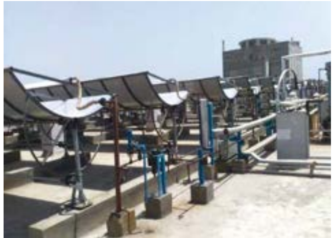
Installation of 615.36 sq. m PTC solar system at AmulFed Dairy, Gandhinagar
