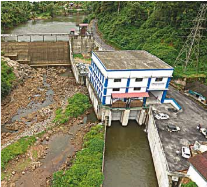
A Small Hydro Project installed at Vellathooval, Kerala
