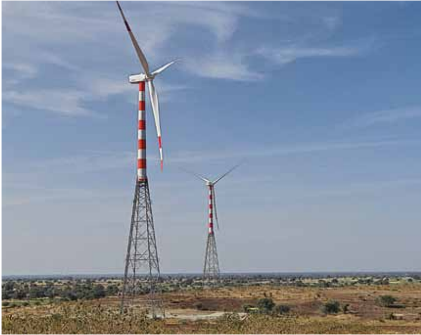
90.3 MW hybrid tower wind farm in Madhya Pradesh
