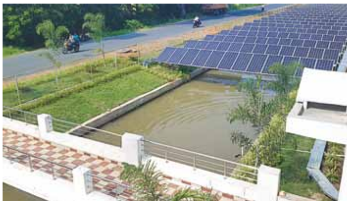
1 MW canal-top solar PV power project commissioned by NREDCAP on Losari Canal, Gollavanitippa, Bhimavaram Rural (M), West Godavari District, Andhra Pradesh.
