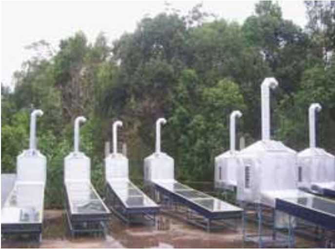
50 kg Solar Turmeric drier at Mizoram, India
