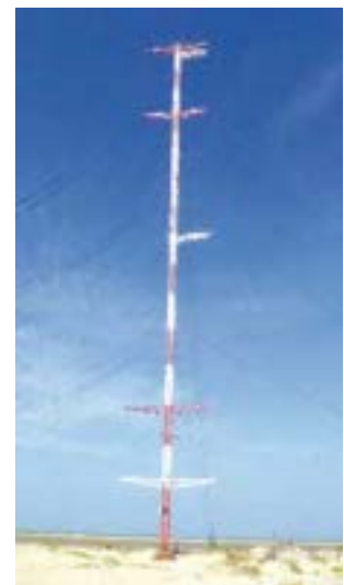
100 m lattice wind mast at Dhanushkodi, Rameshwaram
