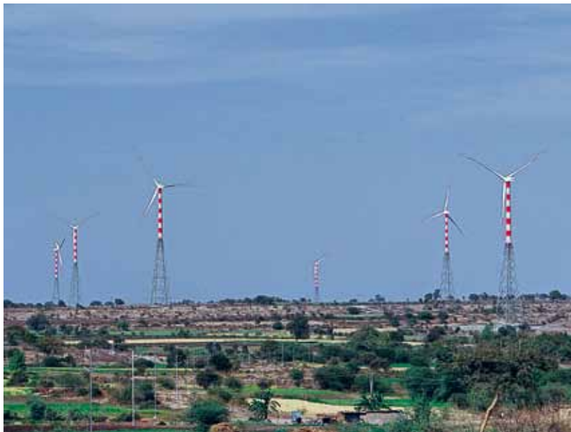
A 90.3 MW Wind Farm in Madhya Pradesh
