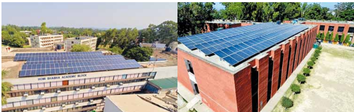
SPV Power Plant at NITTTR Academic Complex (left) and 60 kWp Plant Govt. School Dhanas, Chandigarh (right) under Model Solar Cities Programme
