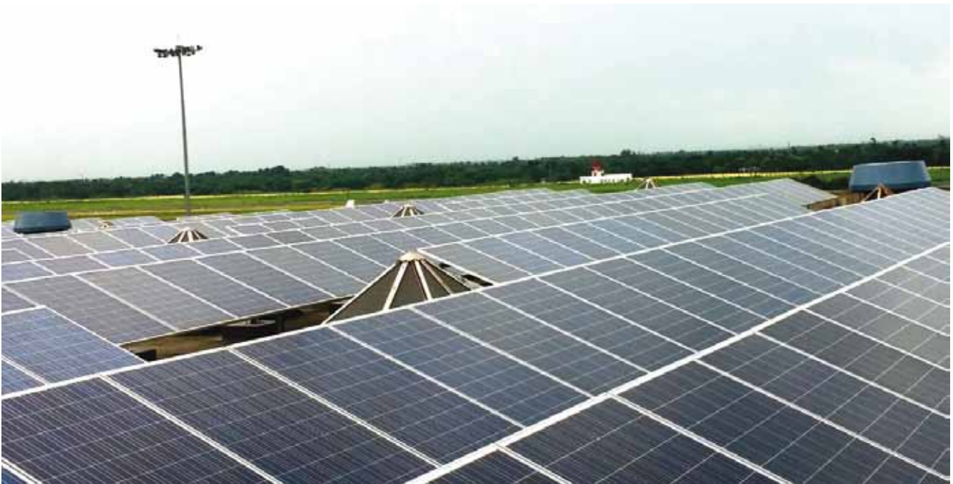
2 MWp grid connected solar rooftop plant at Kolkata Airport, AAI
