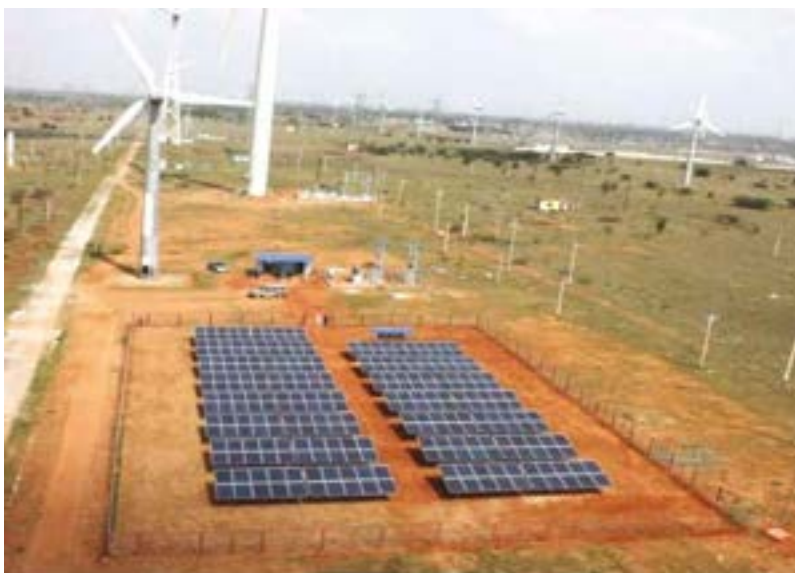
Grid integration of 75 kW solar with 200 kW WEG
