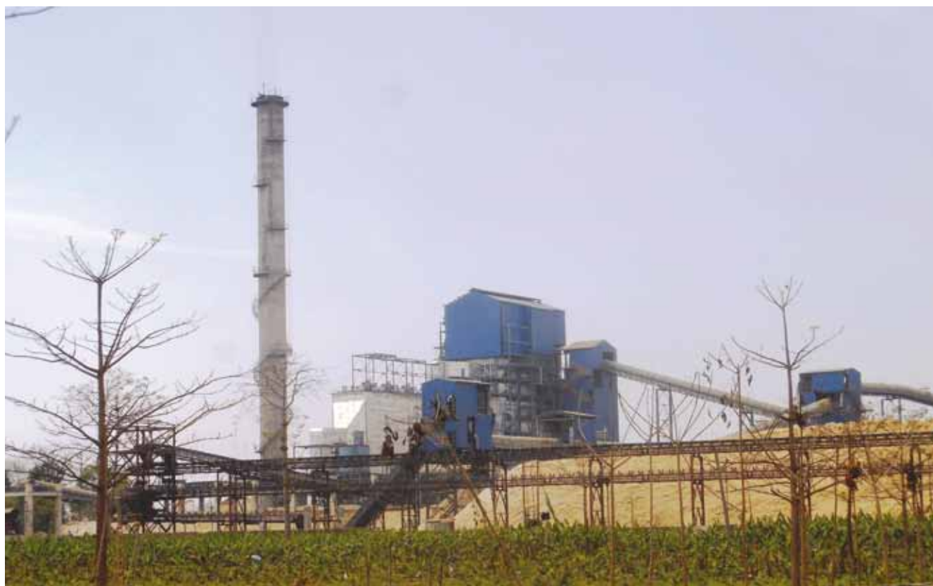
30 MW Cogeneration project of M/s.Gobind Sugar Mills Limited at Lakhimpur Kheri of Uttar Pradesh
