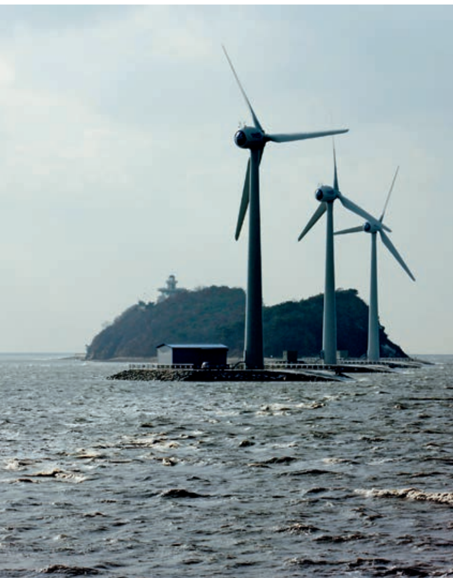
Nue (Silkworm) Island, Kyonggi-do, West Sea of Korean peninsula. Unison 750KW x 3 WTG’s, Commissioned in 2009 © KWEIA
