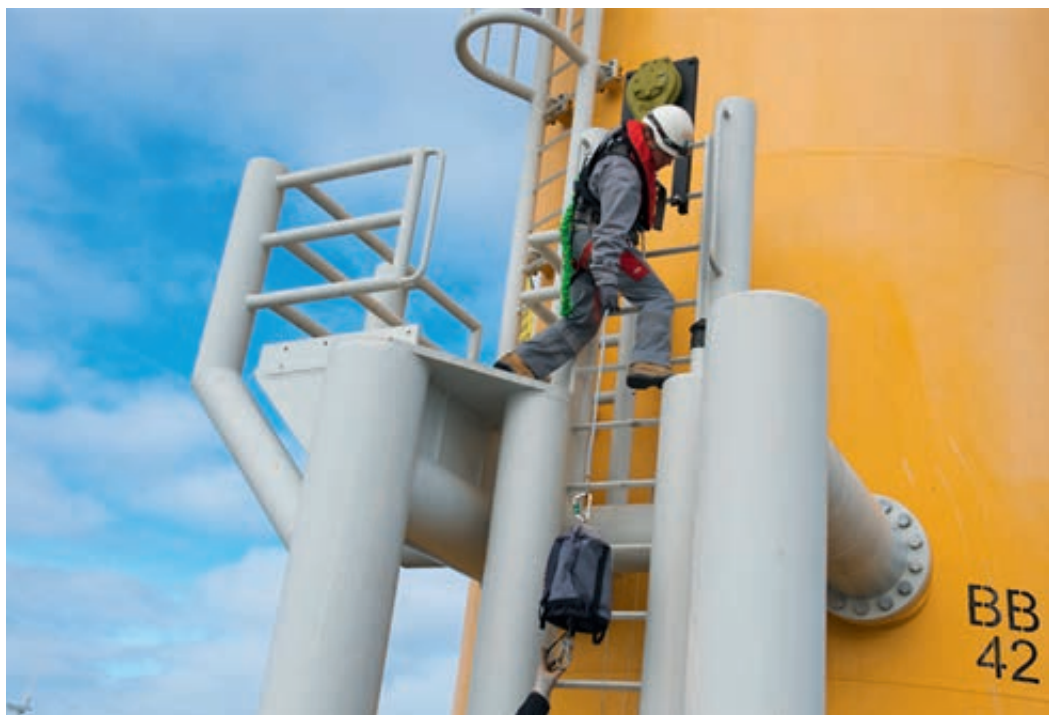
Burbo Bank, Liverpool Bay © RenewableUK
