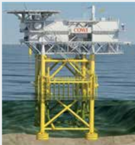
FIGURE 15-6 OFFSHORE SUB STATION FOR A EUROPEAN OFFSHORE WINDFARM
