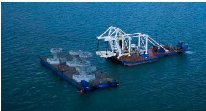
Figure 77 - The bespoke heavy lift vessel Eide 5 lifting GBS foundations at Rødsand
