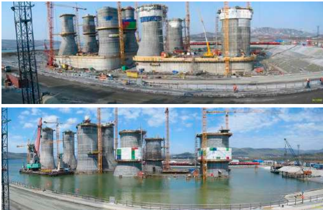
Figure 47 - GBS construction in a dry-dock facility (or graving yard)
