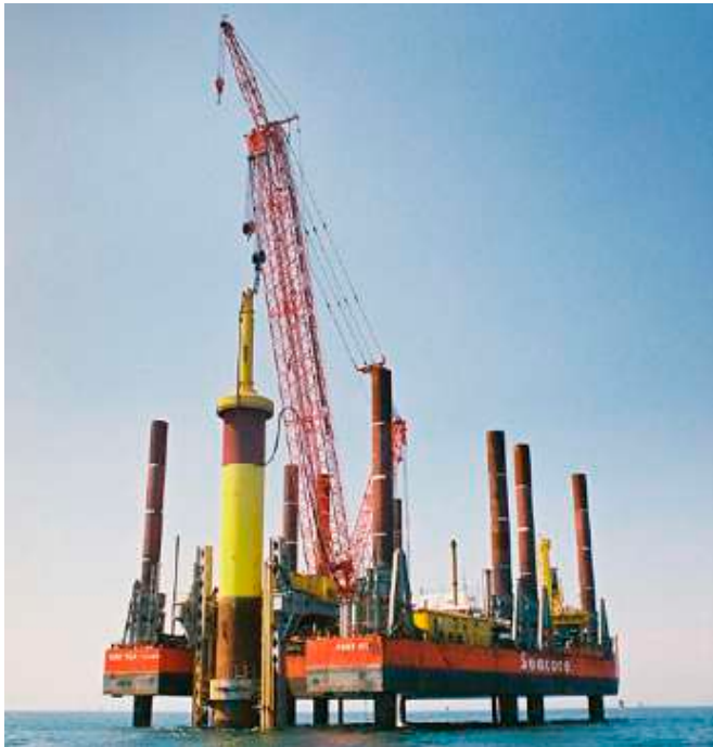
Figure 55 - Fugro Seacore's Excalibur towed jack-up installing a monopile
