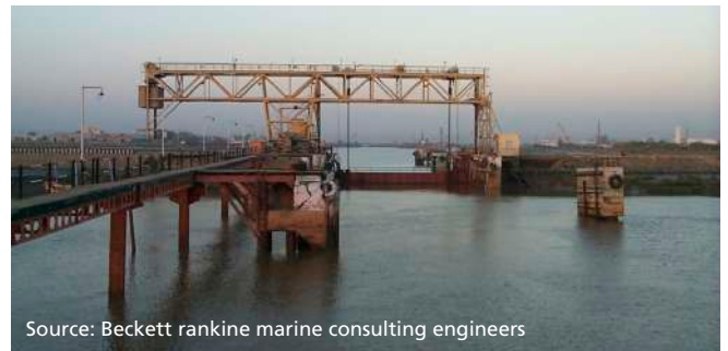
Figure 114 - Bhavnagar Port - lifting gate lowered into position at high tide
