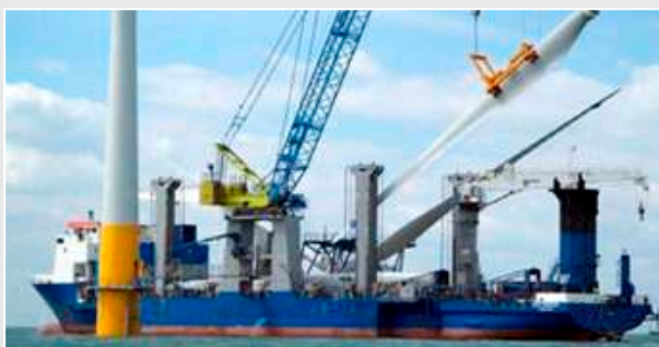
Leg-stabilised crane vessel
