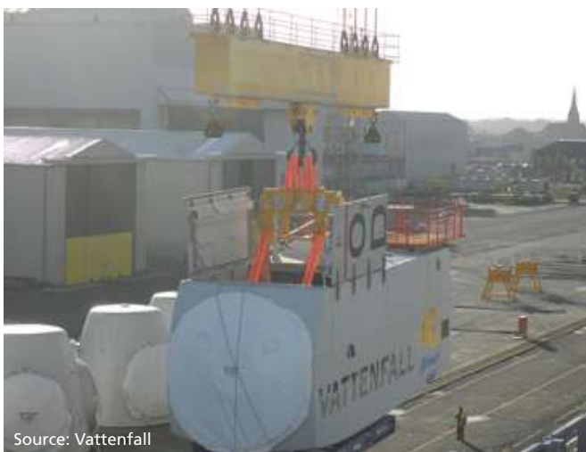
Figure 38 - Port crange nacelle load-out
