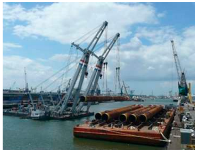
Figure 68 - Transportation of monopiles FND to MAR, using a dumb barge
