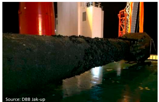
Figure 134 - DBB Jack-up decommissioning operations, removal of offshore masts (left) and associated monopiles (right) on Horns Rev 1 and Horns Rev 2 in Denmark
