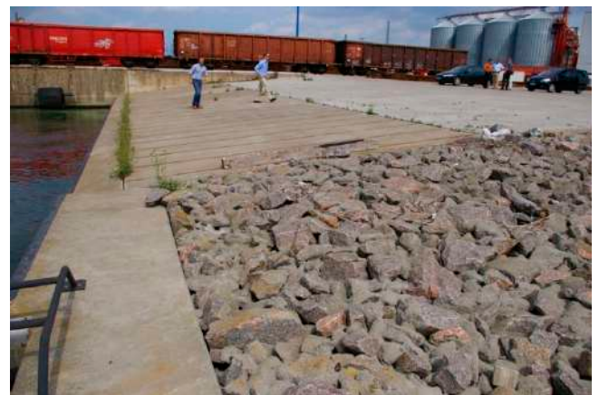
Figure 94 - Concrete ramp, used for RoRo load-outs
