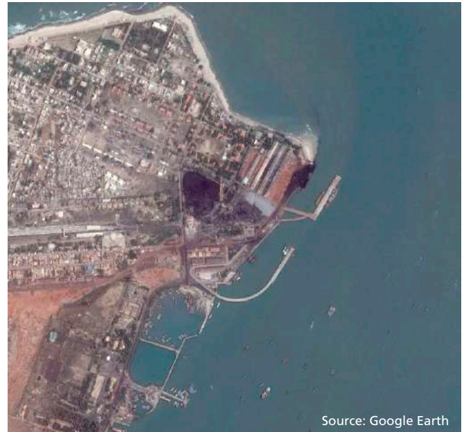
Figure 122 - Port Okha facilities
