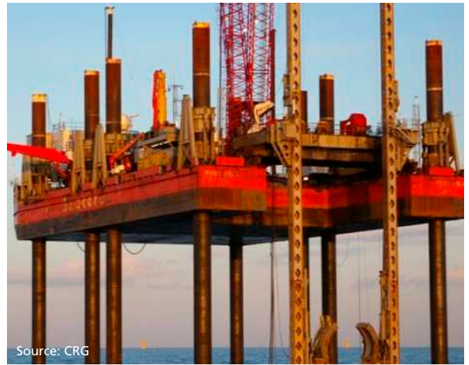
Figure 70 - Piling frame on Excalibur awaiting a floating monopile
