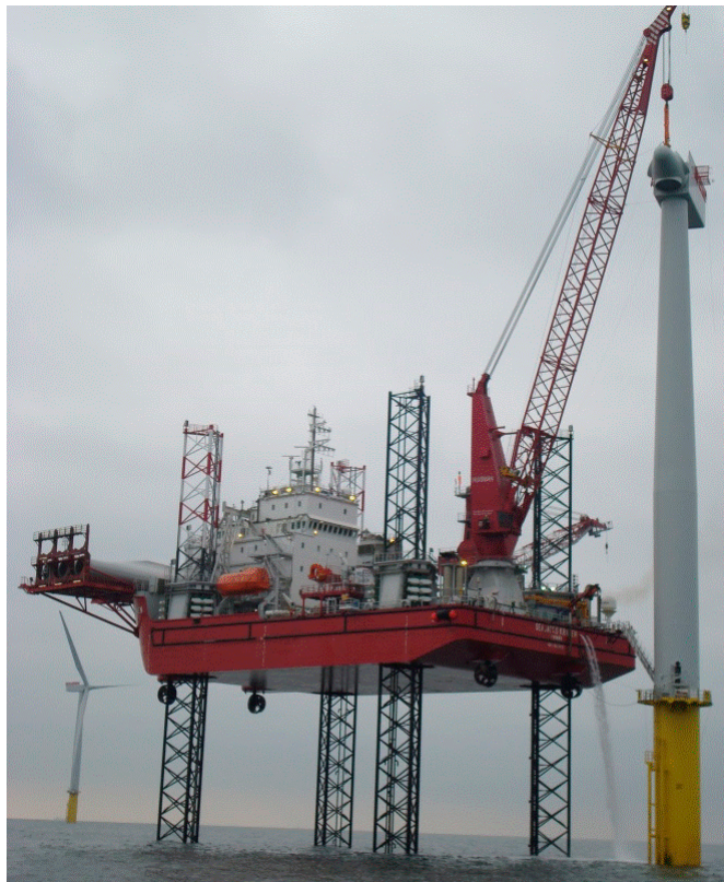
Figure 80 - Wind turbine installation vessels
