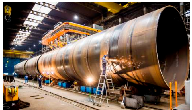
Figure 11 - Jacket fabrication (top) and monopile fabrication (bottom)
