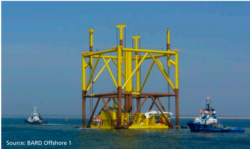
Figure 49 - Self-installing and floating substation designs
