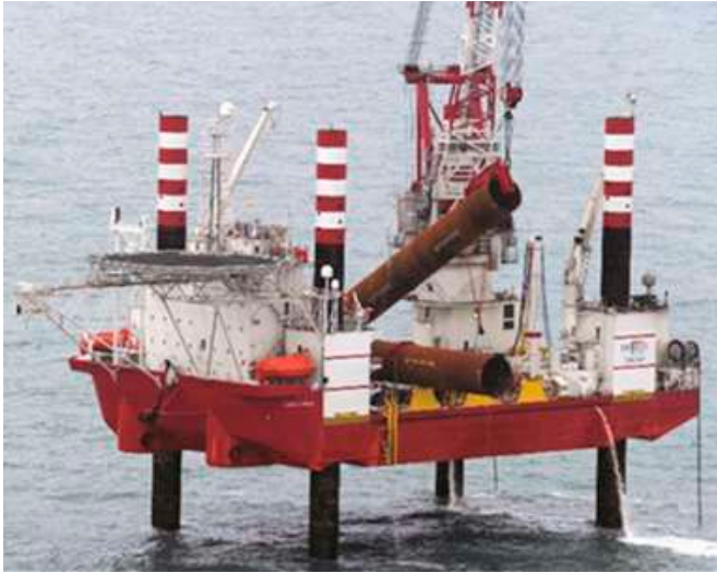
Figure 69 - Jack-up upending a monopile in preparation for piling
