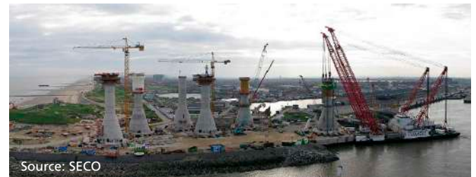
Figure 45 - Construction of GBS on the quay (Thornton Bank)
