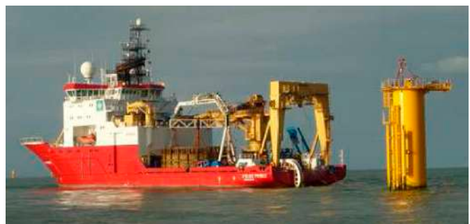
Figure 86 - Inter-array cable laying using an offshore supply vessel
