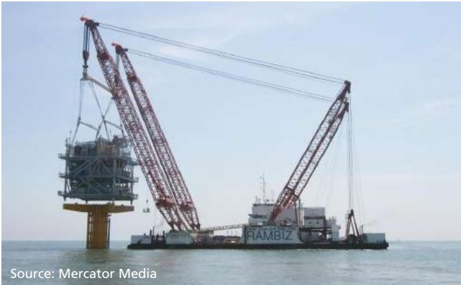
Figure 61 - Rambiz 3, 300 t SHLV installing a substation topside
