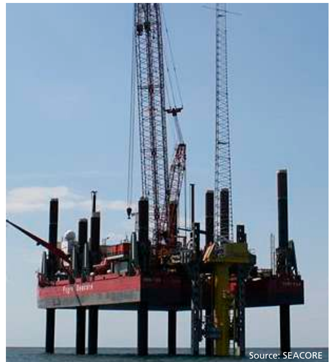
Figure 2 - Offshore met mast installation, UK
