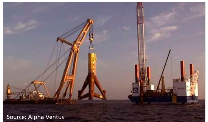
Figure 60 - Sheerleg crane-vessel working in tandem with a jack-up piling vessel
