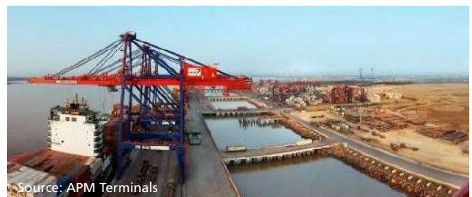
Figure 120 - Vessel berthed in Pipavav
