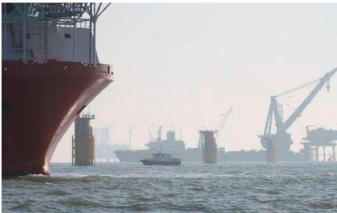
Figure 52 - Busy scene during construction of Thanet OWF
