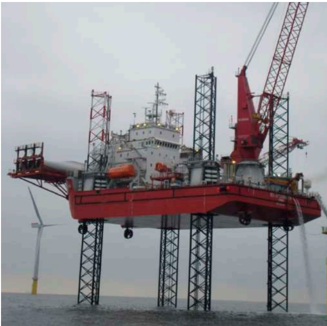
Figure 57 - Gusto MSC NG2500x installing Siemens SWT 3.6 107 at Walney 1 offshore windfarm
