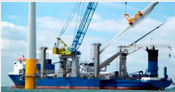
Leg-stabilised crane vessel
