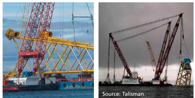
Figure 76 - Rambiz up-ending the leg-sheered jacket at Beatrice
