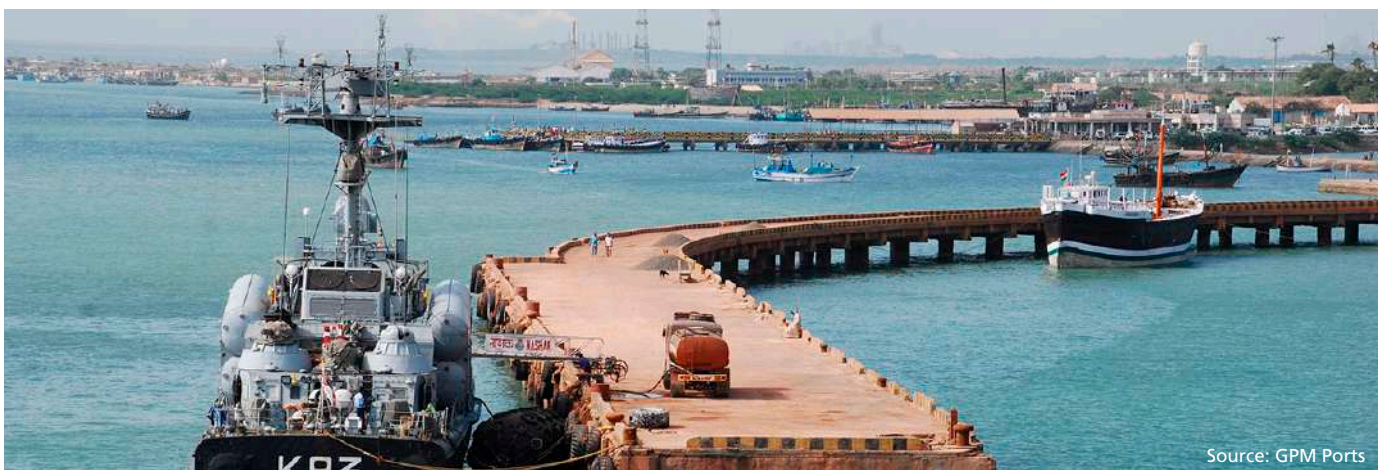
Figure 123 - Okha port berth
