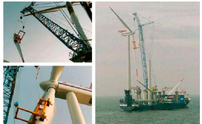
Figure 64 - A2Sea Sea Energy / Sea Power - Leg-stabilised crane vessels
