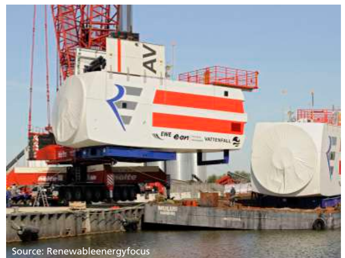
Figure 39 - Crawler crane nacelle load-out
