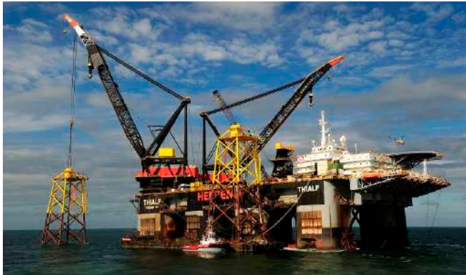
Figure 66 - Jacket installation at Alpha Ventus, by Thialf
