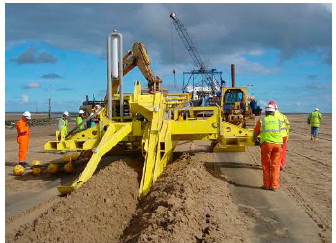
Figure 83 - Subsea cable plough burying cable at the shore
