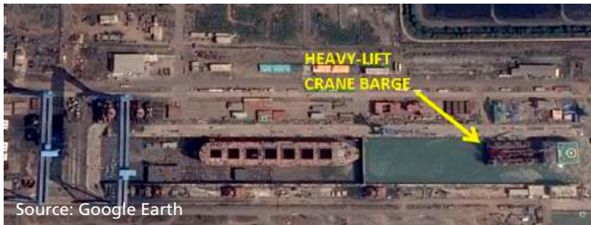
Figure 118 - Pipavav port facilities
