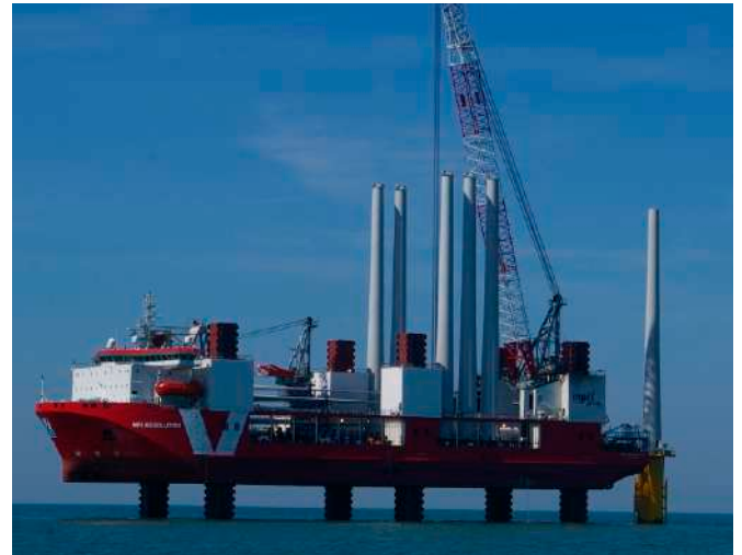
Figure 56 - Wind turbine installation vessel MPI Resolution at Thanet OWF
