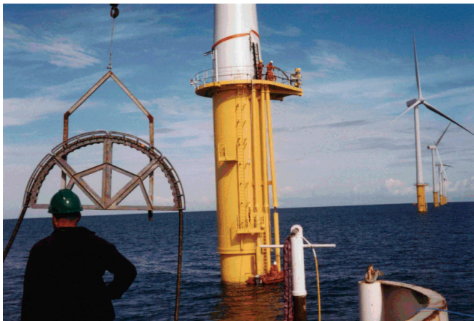
Figure 84 - Cable installation adjacent to a wind turbine
