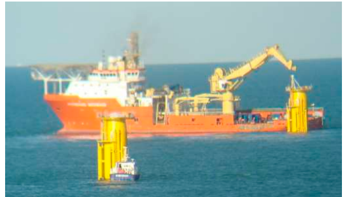
Figure 65 - DP2 offshore construction support vessel installs array cables - Normand Mermaid
