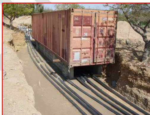
Figure 57 Onshore cable jointing container - arrangement
