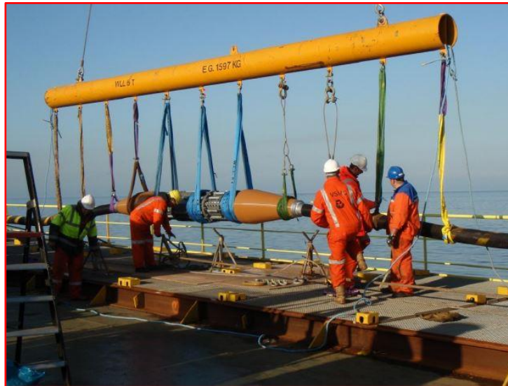
Figure 19 HV cable joint over boarding from cable jointing barge
