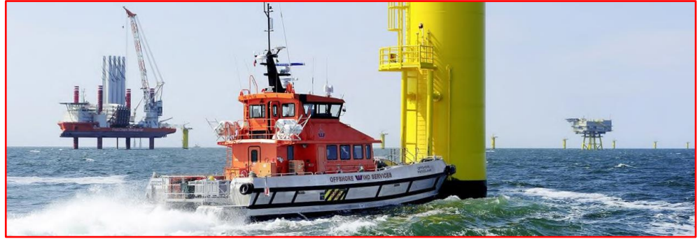
Figure 50 Transfer from CTV to WTG monopile
