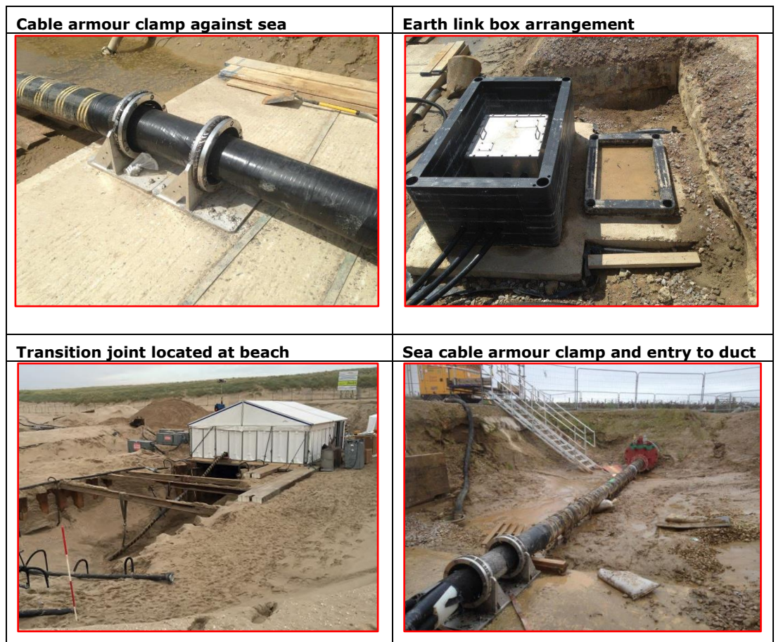
Figure 48 Pictures of transition joint bay (TJB)
