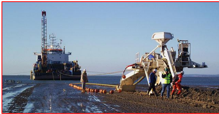
Figure 38 Cable ploughing operation - low tide at beach
