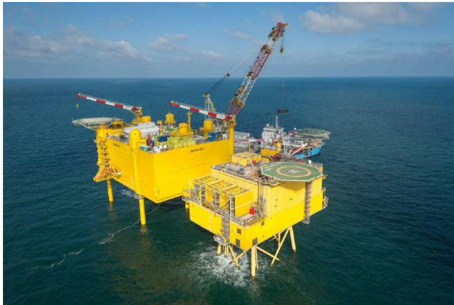
Figure 30: Borwin Alpha (400MW) and Borwin Beta (800MW) installed side-by-side [31]
