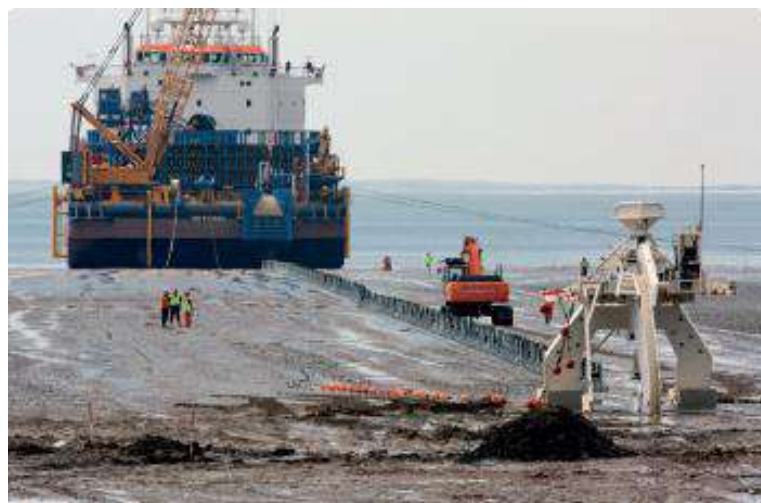
Figure 33: Cable barge and plough making landfall [31]
