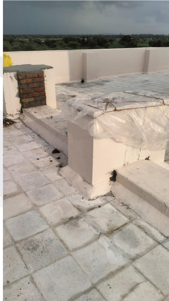
Sealing Expansion Joint
