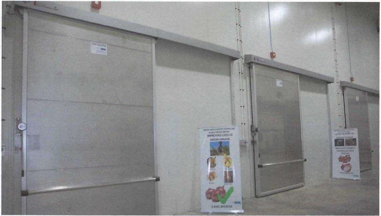
Onion-specific cold storage developed by BARC for preservation trials and technology demonstrations at the KRUSHAK food irradiation facility in Lasalgaon, Nashik
