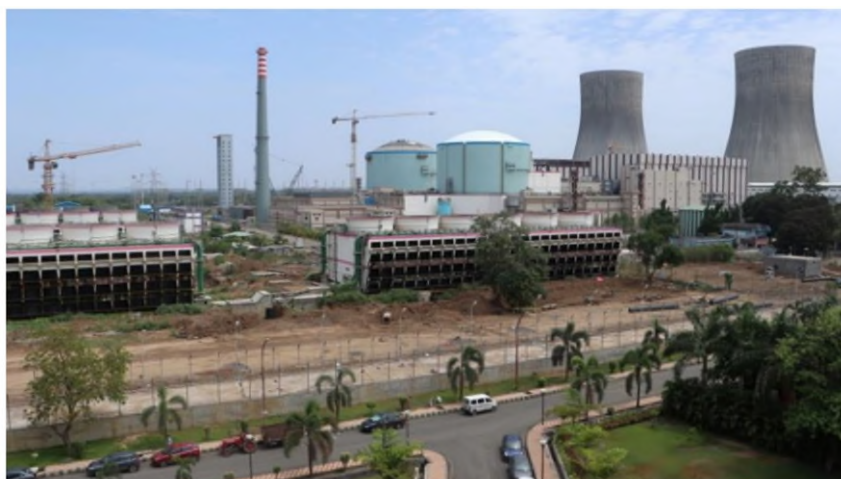
Kakrapar Nuclear power Plant
