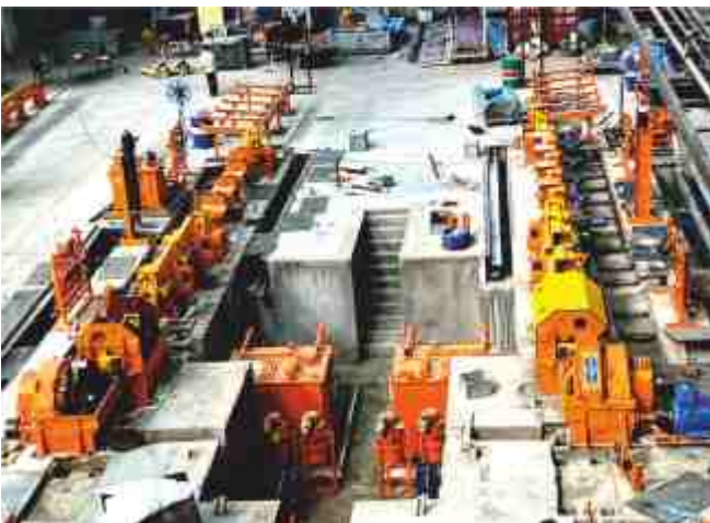
32mm CRTM/ Pilger Mill – Under installation
