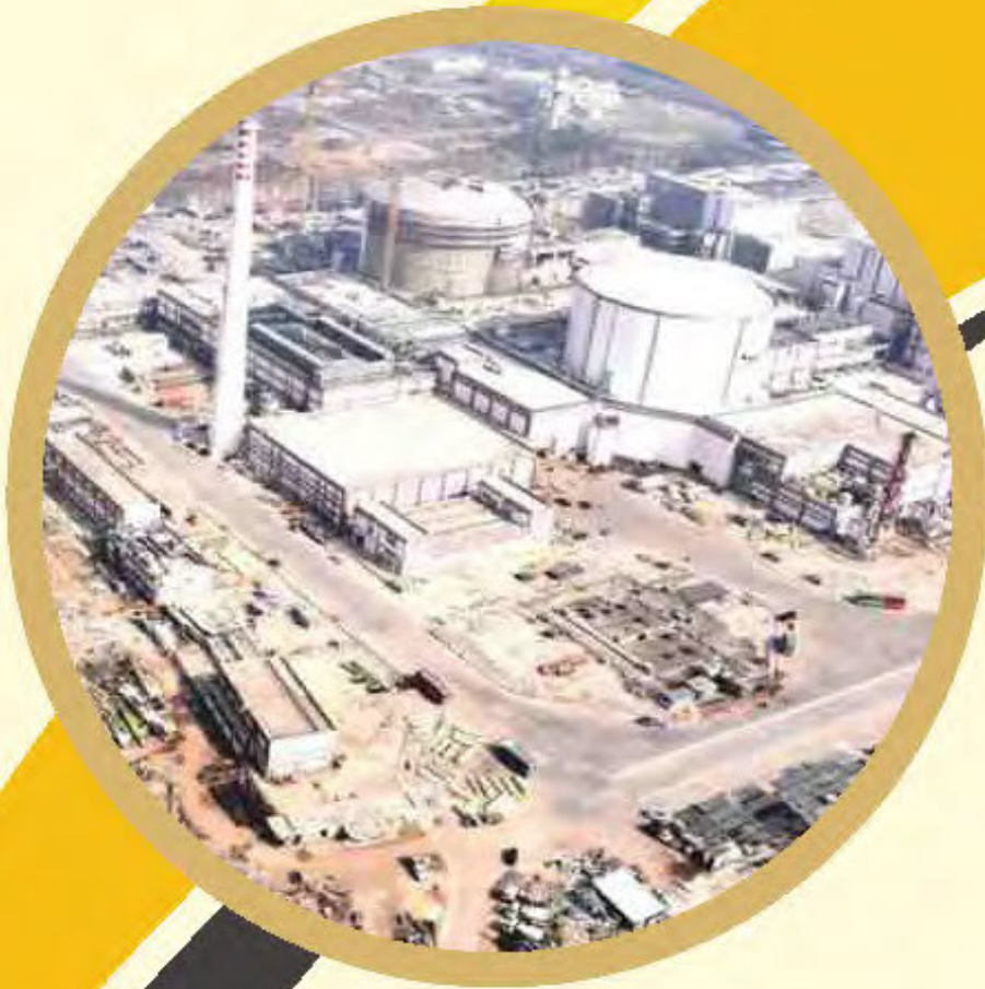
Site View of Rajasthan Atomic Power Project RAPP-7&8
