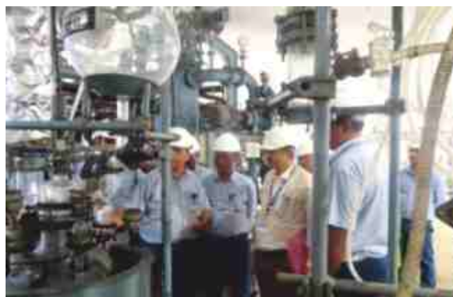
CC-6 production unit at HWBF, Talcher
