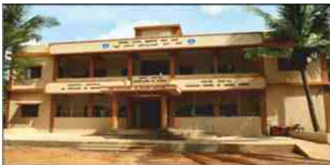
Construction of Government Higher Primary School, Bare, Uttar Kannada District, Karnataka
