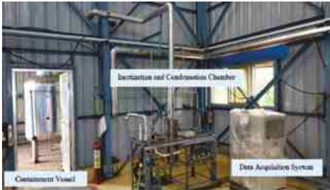
Alternate Hydrogen and Steam Concentration Monitoring System (AHSCMS)
