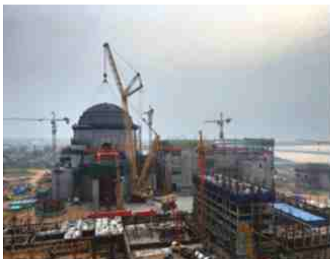
View of IC Dome Liner erection in Reactor Building-3
