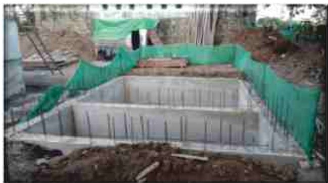
Construction of Sewage Treatment Plant by HWB for Surat Municipal Corporation
