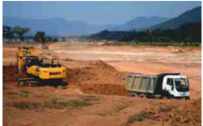
Excavation works of Kaiga-5&6
