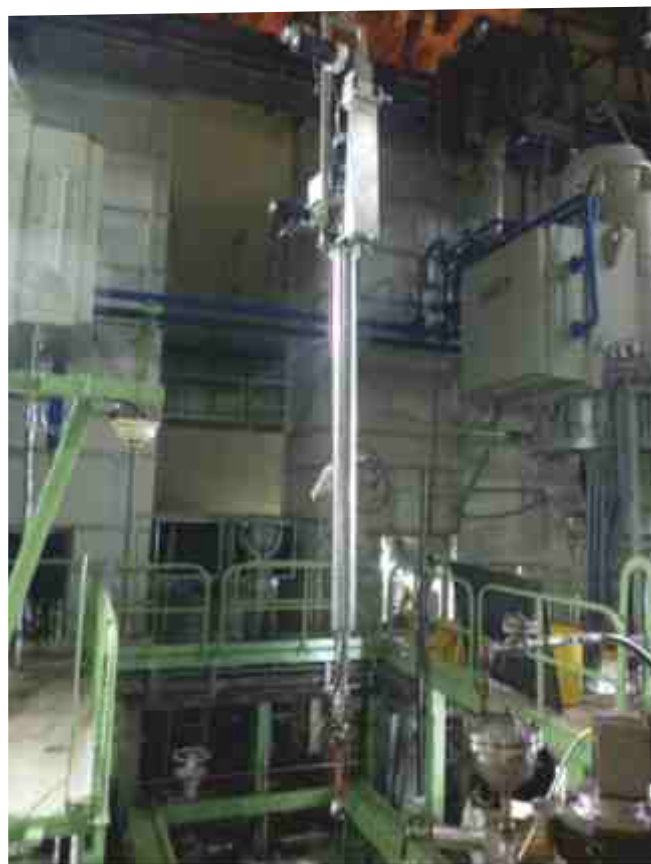
HBOSS Welding Manipulator Being Lowered to Exact Location
