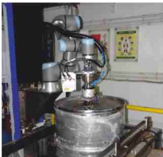
The Automatic Drum Handling System of BARC for deployment in operations involving remote filling and emptying of D 2 O storage drums
