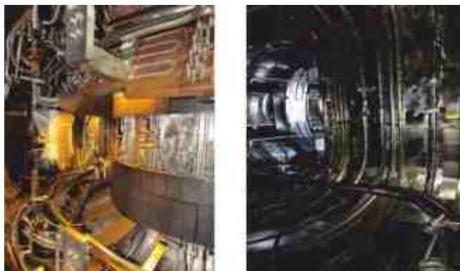
Inside view of SST-1 vacuum vessel before and after PFCs removal
