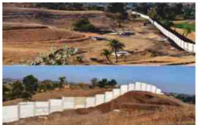
View of Mahi Banswara Plant Boundary Wall
