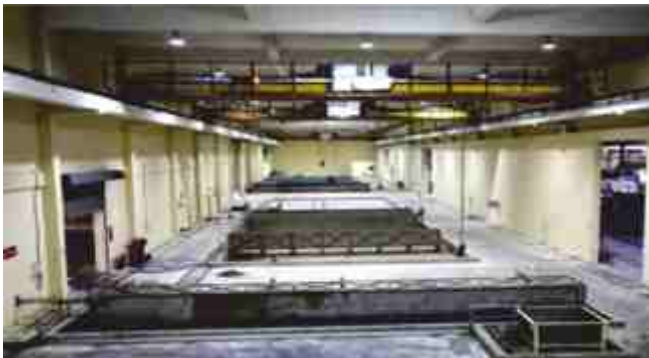
Establishment of New Degreasing and pickling Section at ZFP
