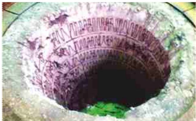
Old 200kW Furnace
