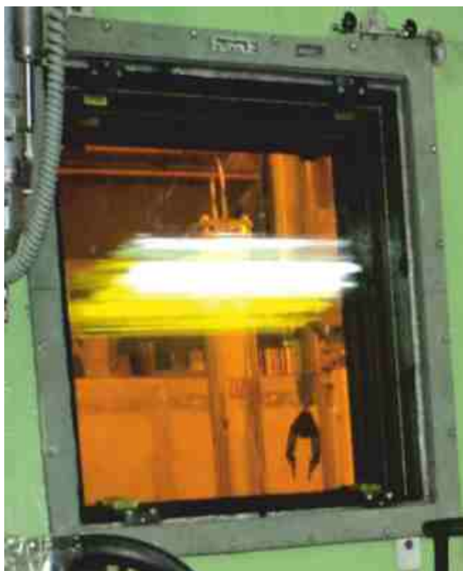
Newly Commissioned Radiation Shielding Window of Integrated Nuclear Recycle plant (INRP) in Tarapur
