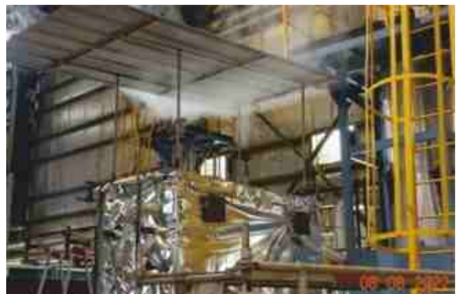
Calandria Vault Test Facility
