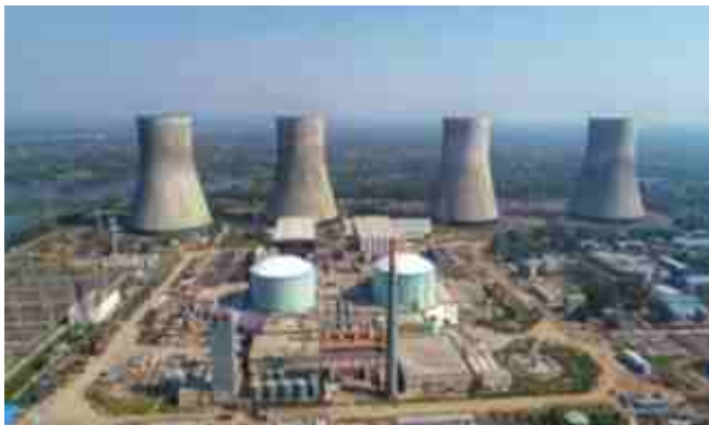
Main Plant Construction area view – KAPP-3&4
