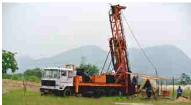
Departmental drilling unit at in field area of Eastern Region
