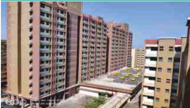
HBNI Hostel M1 M2 Building
