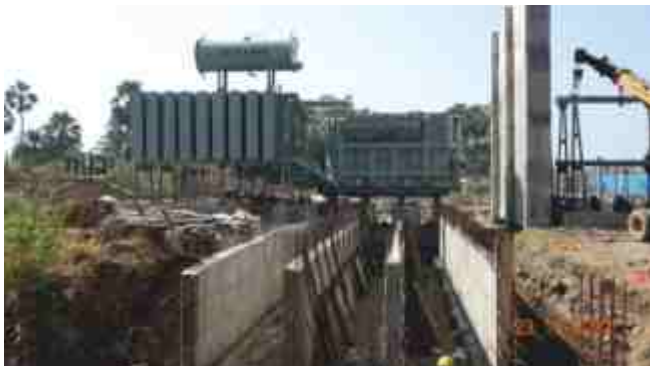
50 MVA Transformers Erection in Progress
