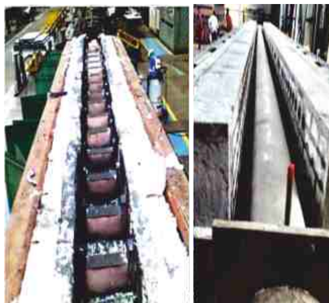
Internal View of Old Furnace (left) Internal View of New Furnace (right)
