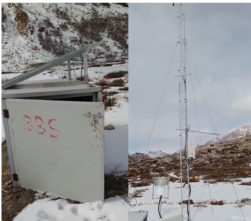
Figure 1. Photograph of the inspection of the Automatic Weather Station at Bhojwasa on 9 th February 2026 by the watch and ward team, displaying data under harsh weather conditions.
