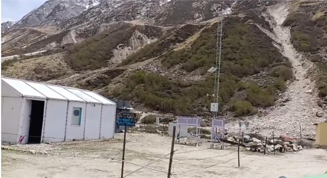
Figure 2. Photograph showing the instrument location and the temporary fencing constructed to protect the instruments at Bhojwasa.
