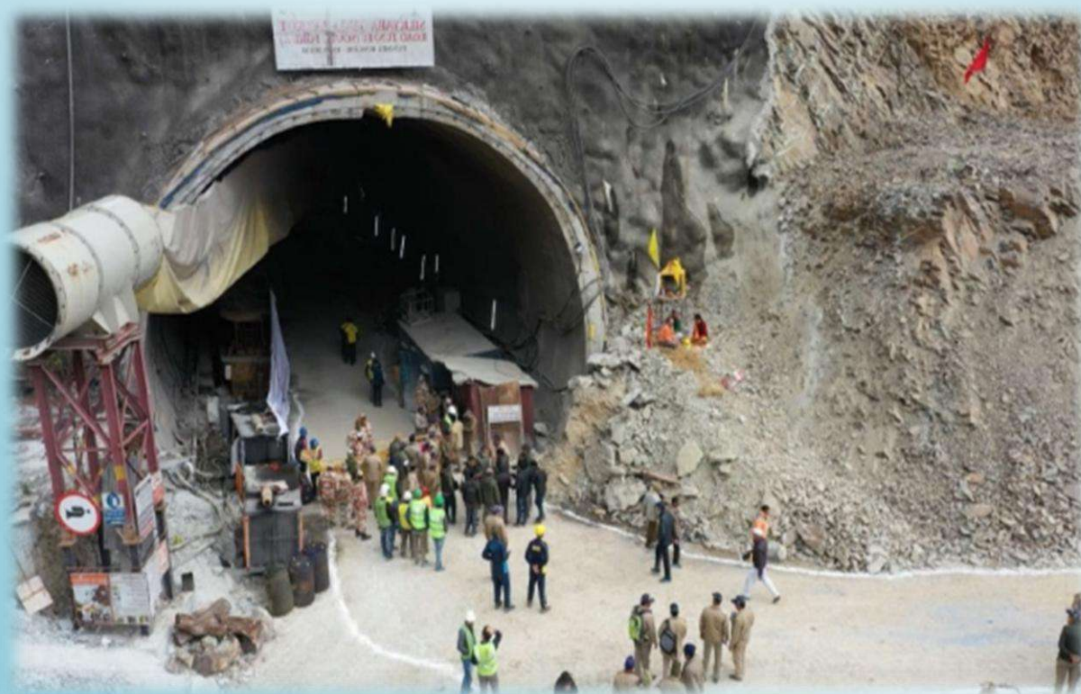
Portal of Silkiyara Tunnel
