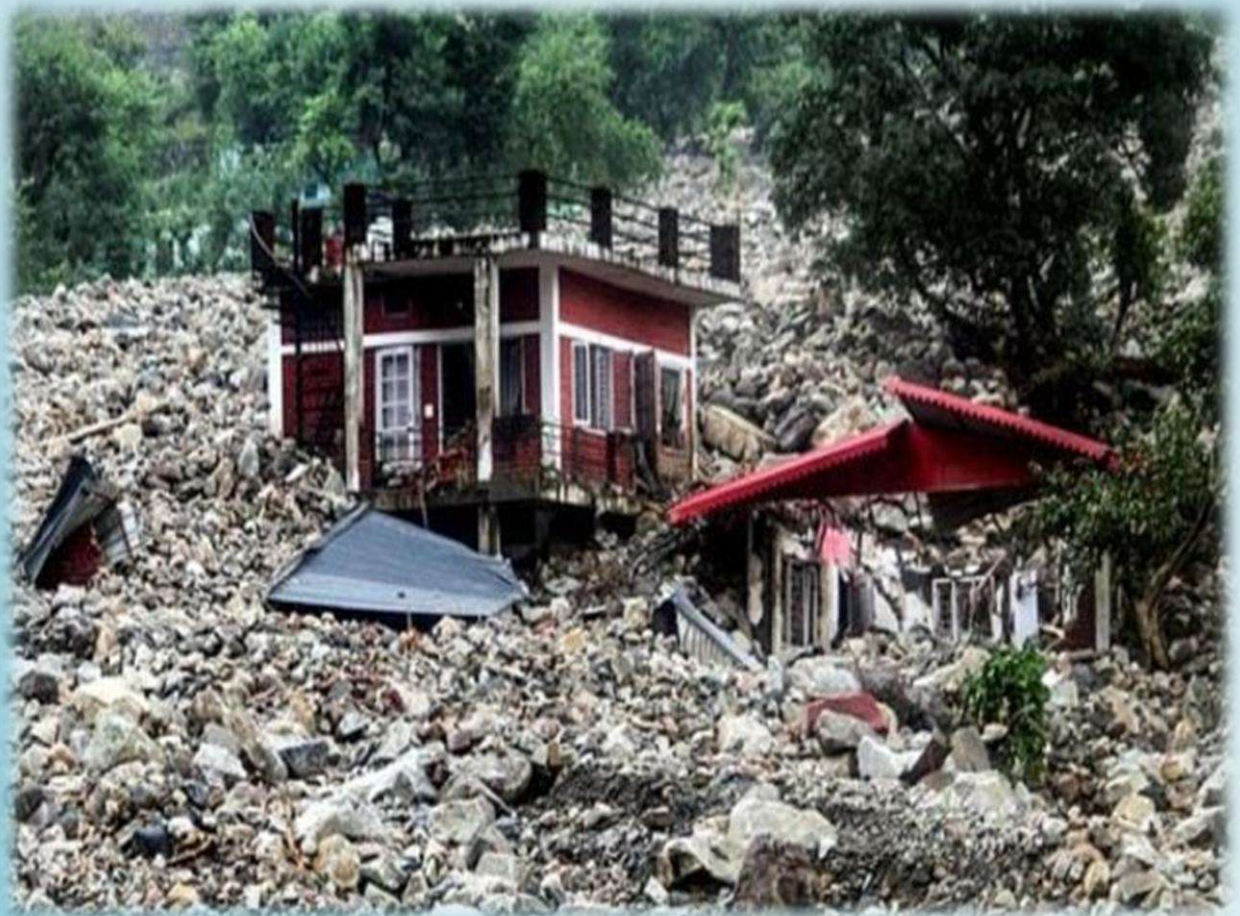
Ruined Building after cloudburst at Sahastradhara in Dehradun
