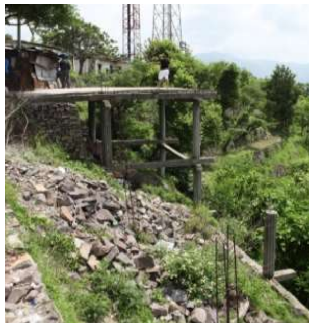
2) Constructing the Plinth level at steep slope- use of RCC Beams and Columns
