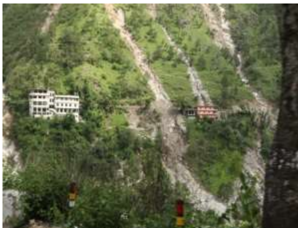
1) Multi-floor Building in the high land slide zone,
