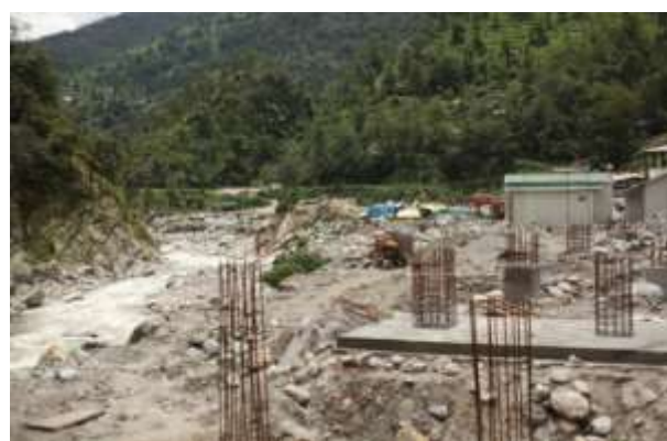
4) Erecting RCC Structure at River Bed
