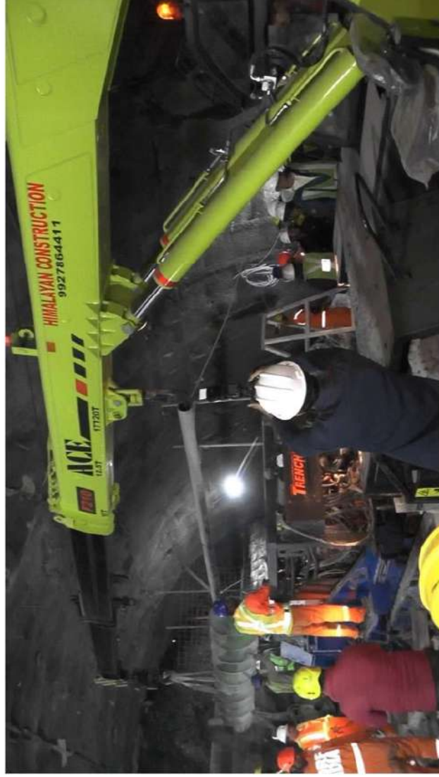
In Figure 10, dated December 14, 2023, the Auger Machine Blade has been positioned to facilitate horizontal drillings, marking a significant step in the operational process.
