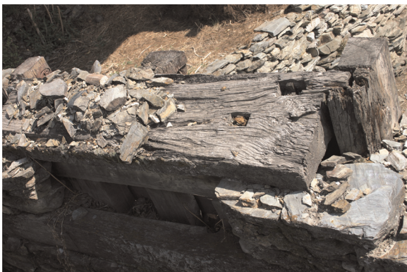
Fig. 8. Photograph showing housed and nailed joints used for fixing the wooden components of traditional houses.
