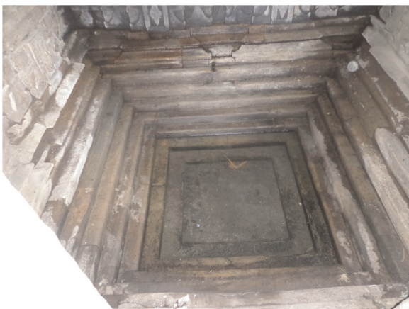
Fig. 3. View of stone lined stepped architecture of shallow dug well, naula in local parlance.
