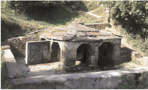
Fig. 2. View of traditional shallow dug well, naula in local parlance.
