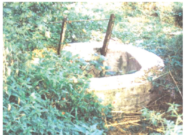
Fig. 5. View of brick lined deep dugwell at Almora.
