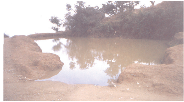
Fig. 6. View of traditional recharge pits, chal and khal .
