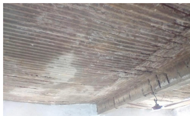
Fig. 5. Poorly constructed roof with clearly visible reinforcement at Government Primary School Mhalchora in Bageshwar district.
