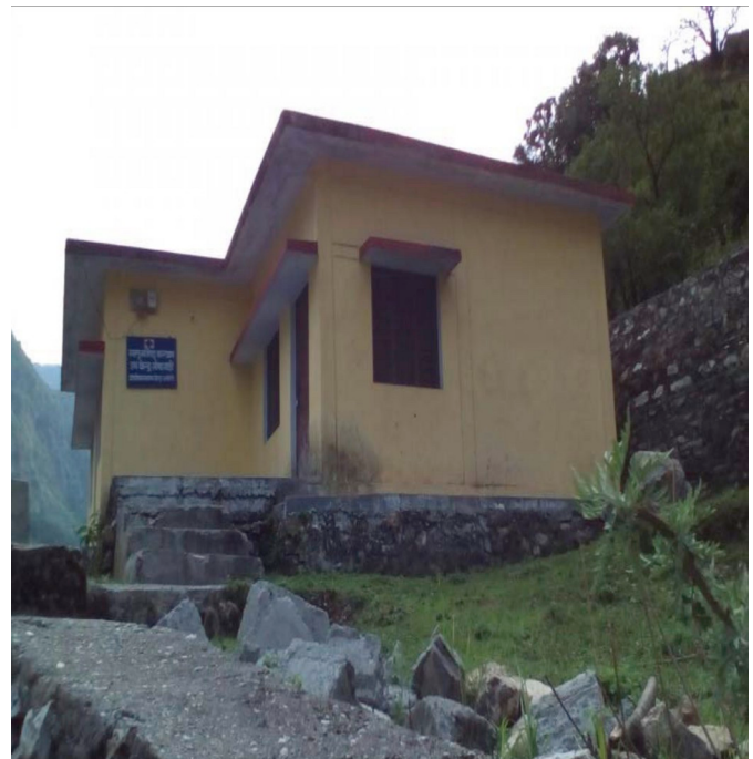
Fig. 7. Re-entrant corners in Upkendra, Gauna, Dasholi in Chamoli district.
