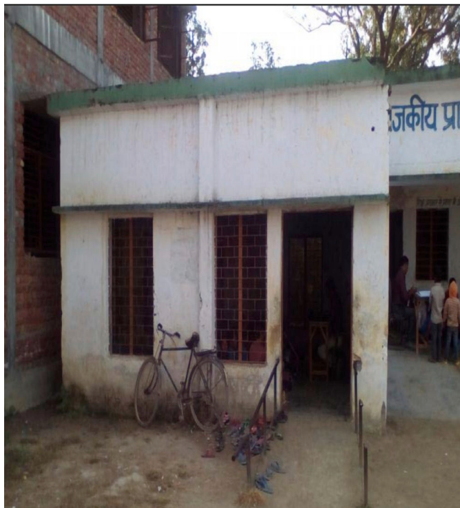
Fig. 9. Government Primary School, Bajpur in Udham Singh Nagar district is vulnerable to pounding during seismic shaking.
