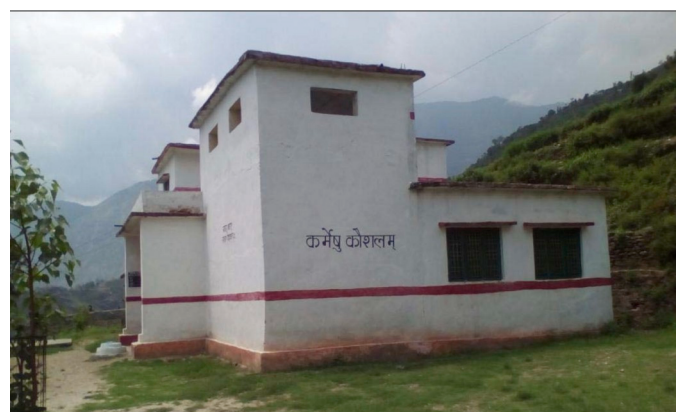
Fig. 8. Re-entrant corners Upper Primary School Balidhar, Dasholi in Chamoli district.
