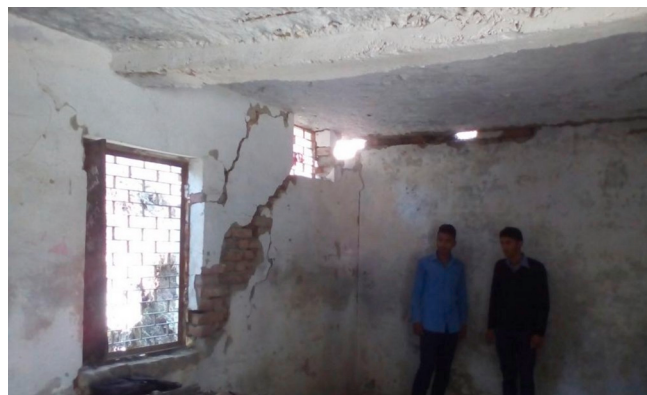
Fig. 4. Wide shear cracks in masonry wall of Government Inter College, Pitrdhar (Rudrapur district) together with poorly constructed beam of non-uniform shape showing deflection.
