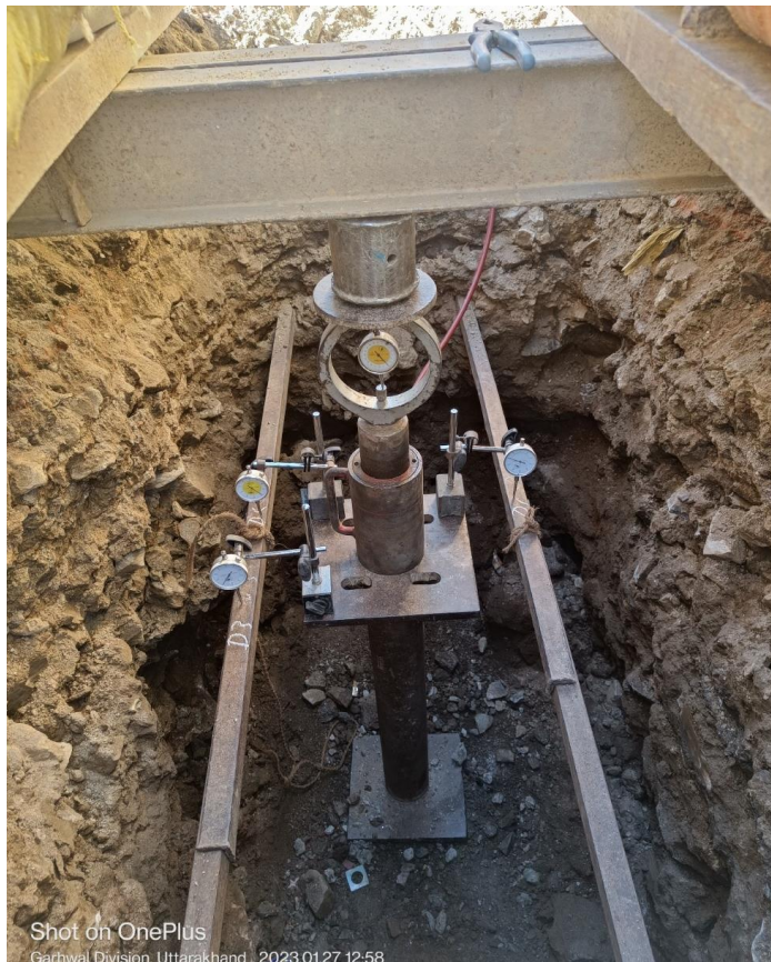
Fig. P6: Plate Load Test, Near Narsingh Mandir (Ward 3)
