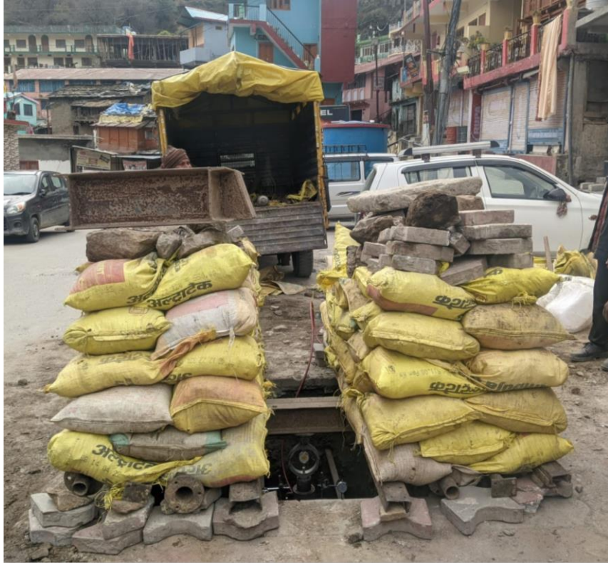
Fig. P5: Plate Load Test, Near Narsingh Mandir (Ward 3)
