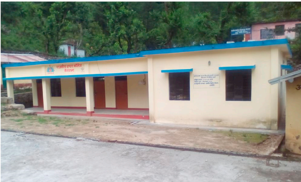
Fig. 12. Single storeyed Government Inter Collage at Bairangana in Chamoli district having RCC slab as the roofing material and exhibiting re-entrant corner.
