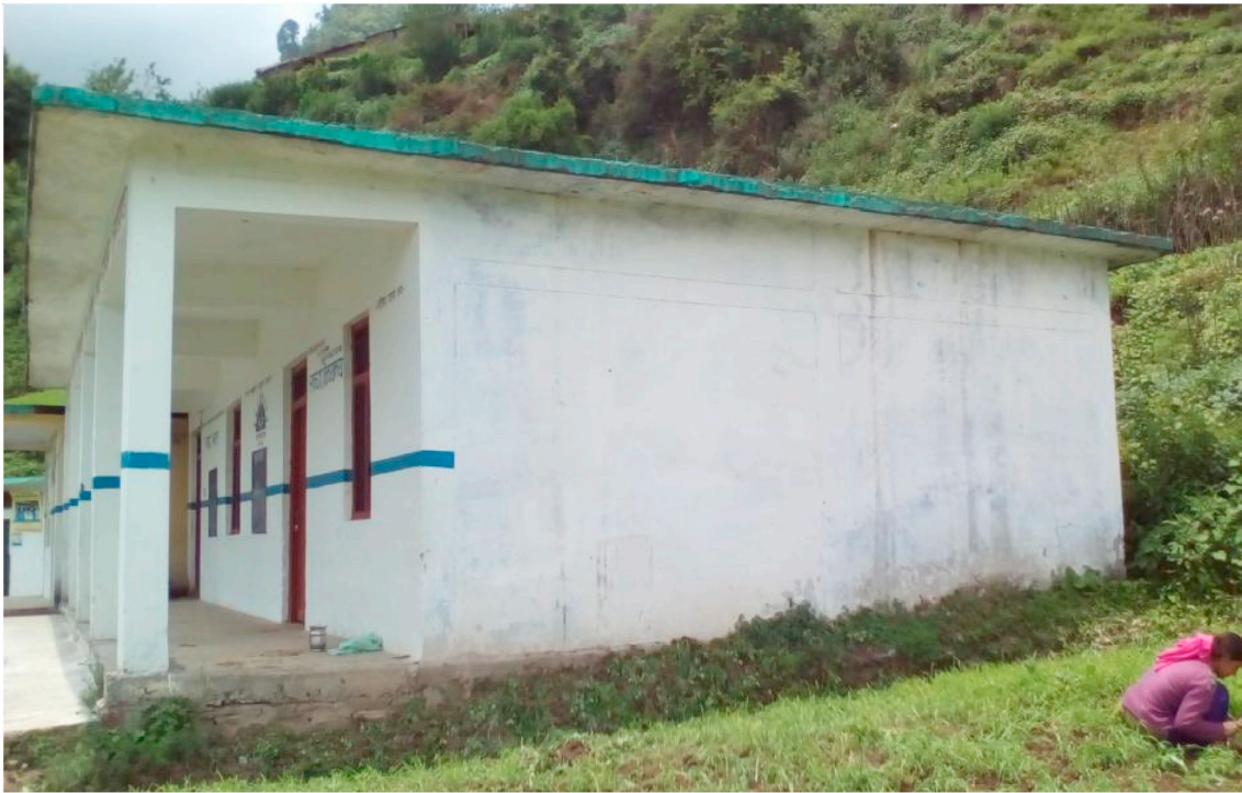
Fig. 6. Government Inter Collage at Trijugi Narayan in Rudraprayag district having RCC slab as the roof and built over soft soil.
