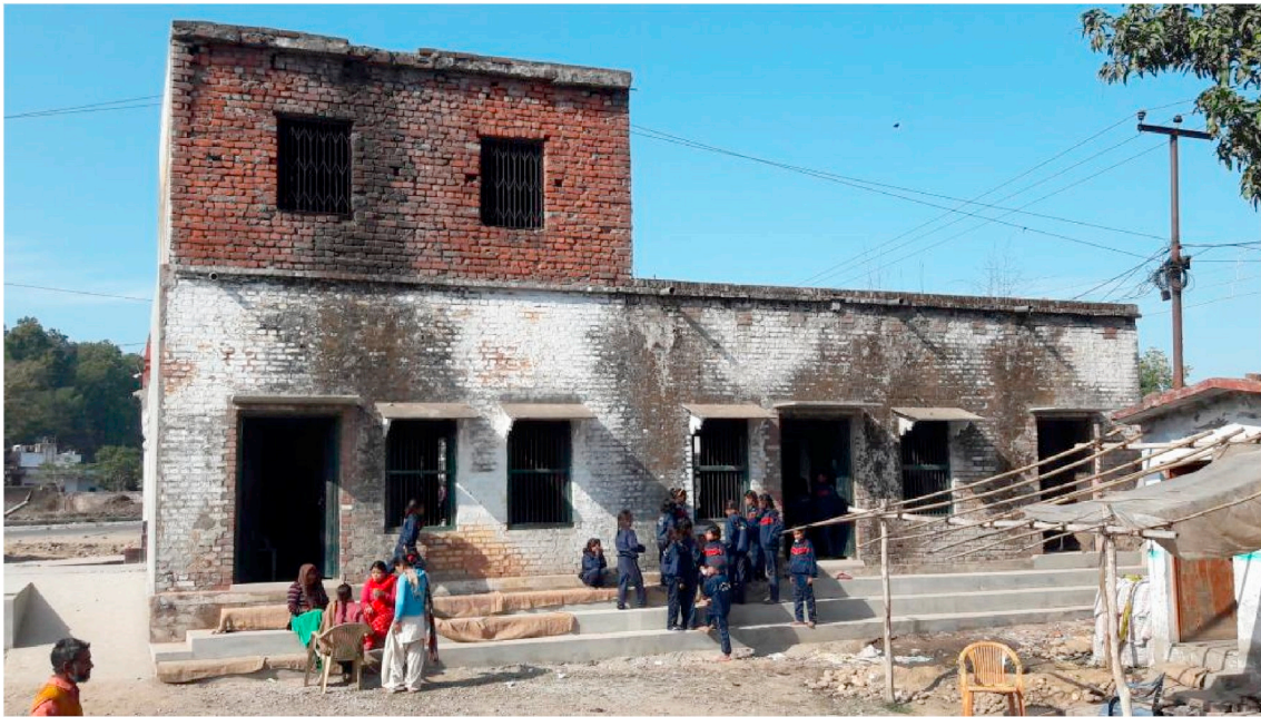
Fig. 8. Primary School at Motichoor in Dehradun representing a non-engineered double storeyed masonry structure.
