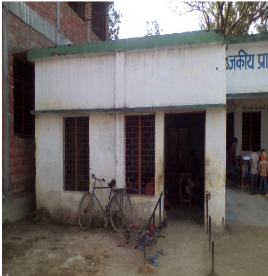
Fig. 14. Government Primary School at Bajpur in Udham Singh Nagar district; vulnerable to pounding during seismic shaking.
