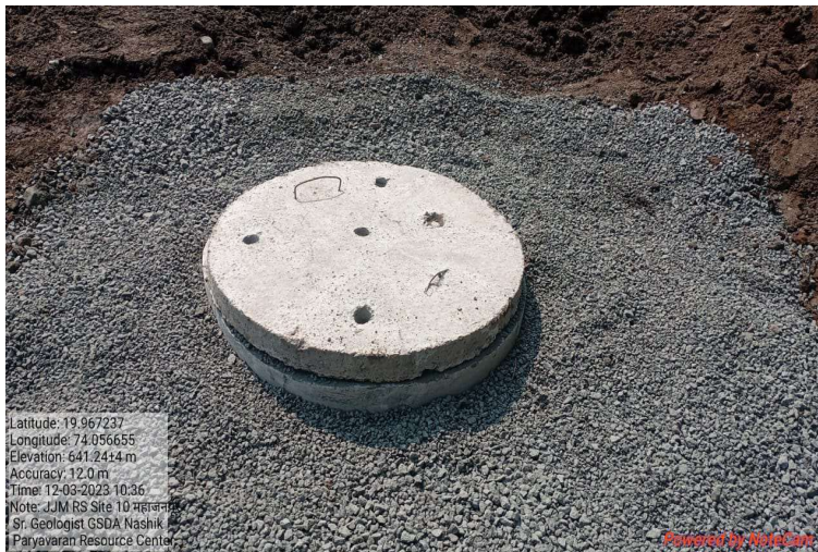
Final Recharge Shaft
