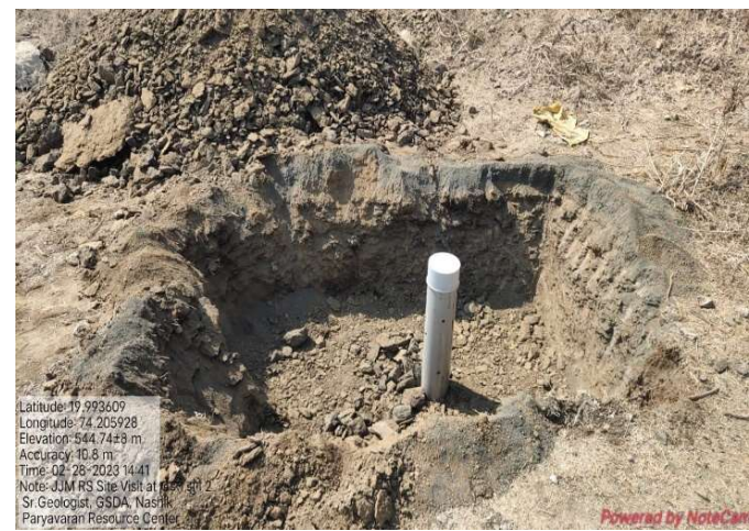
Excavation of Pit
