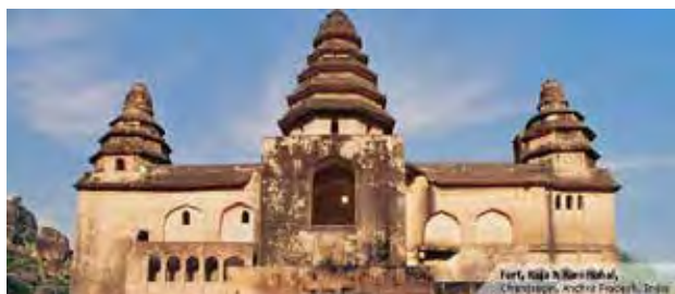
Chandragiri Fort and Palace
