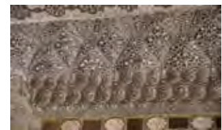
Work on Diwan-e-Khas, Red Fort
