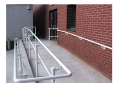
Handrails should be circular in section with diameter of 40-45 mm; at least 45 mm clear of the surface to which they are attached; at the height of 850 – 900 mm from the floor, extended by at least 300 mm beyond the head and foot of the flight or ramp.
