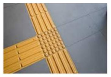
Tactile flooring is a supportive infrastructure with a slip-resistant feature. It helps visually impaired to navigate safely and independently through sidewalks and staircases. It helps prevent accidents and facilitates access.
