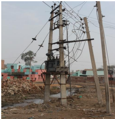
Image 3.19 – Poorly maintained Transformer placed in wetland, Amboli, Jhajjar
