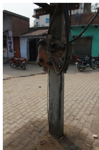
Image 3.14 – Low level live wires as a fuse box, Village Malab, District Mewat [Nuh]
