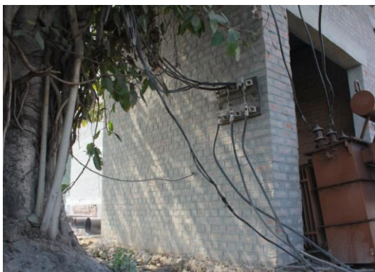
Image 3.17 – Poorly Maintained transformer site, Jhajjar Urban
