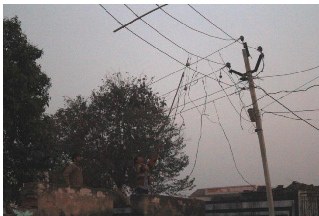
Image 3.16 – Citizens using electricity illegally by clinching metal hooks over main line - Village Parbhuwala, Hisar
