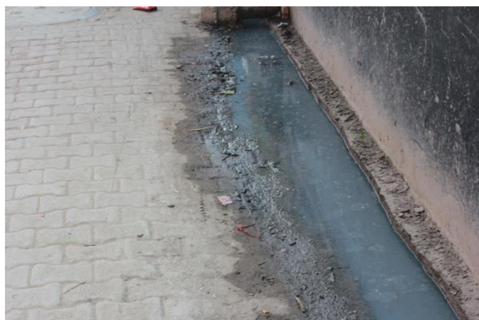
Image 4.15 – The flooding open drain line in Ward No. 14, District Jhajjar
