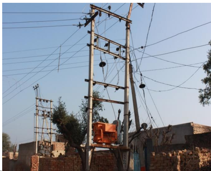
Image 3.13 – Poor state of transformer, Village Chilkani Dhab, Sirsa
