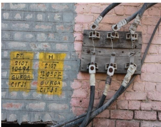
Image 3.15 – Poorly maintained and open fuse assembly at Jhajjar
