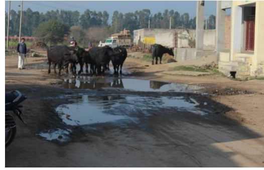
Image 3.8 – Water Logging on road caused because of leakage in water pipeline, Shankarpura, Hisar
