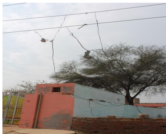
Image 3.12 – Illegal use of electricity, a common site
