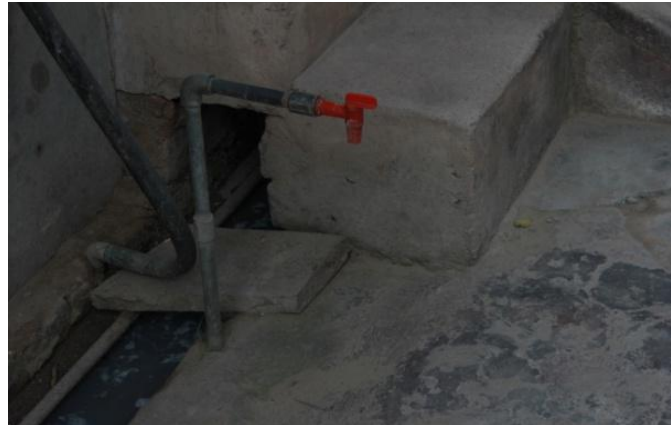
Image 3.10 - Drinking water emerged from sewer line, Ward No. 18, Jhajjar
