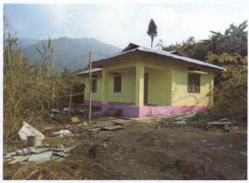
T-IV - 1 No. (Brick work)
