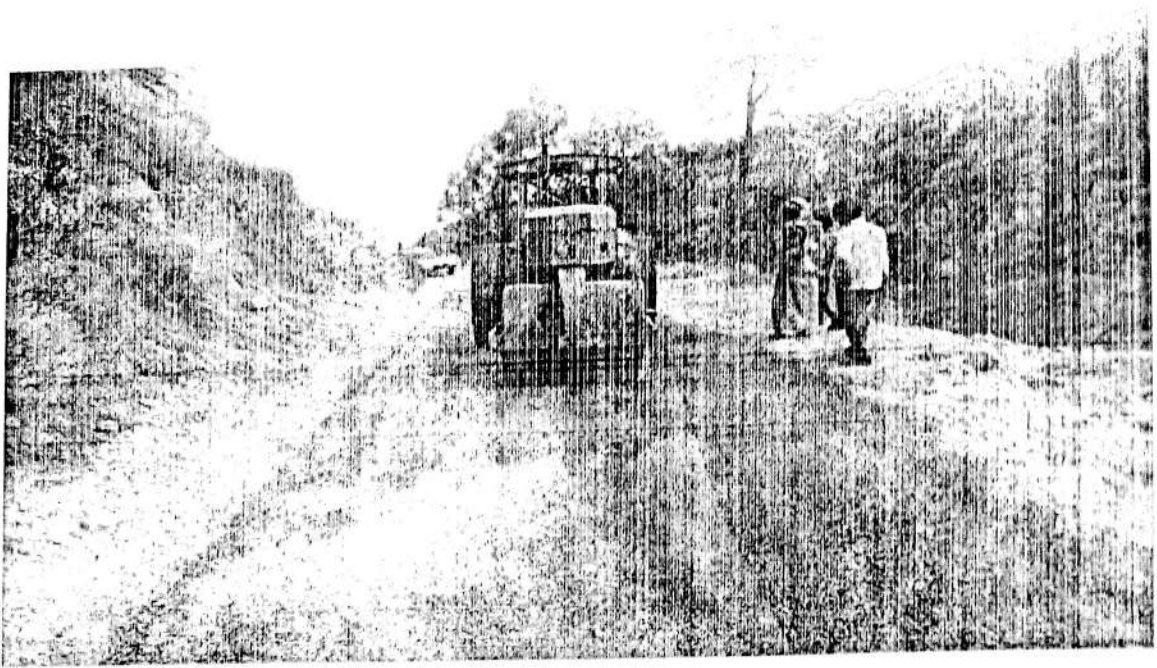
Photo 11: Compaction of Liquid Seal on Premix Carpet
