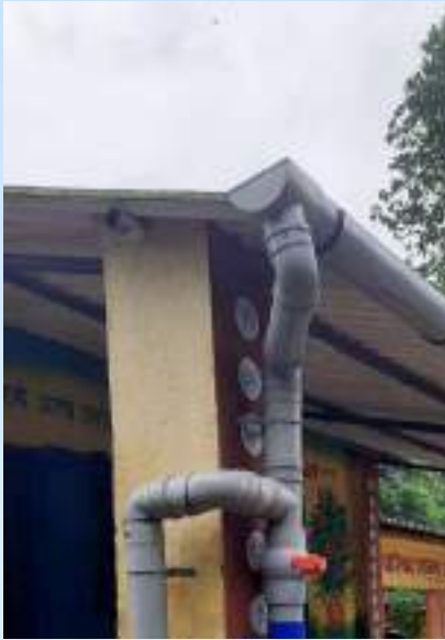
A system of pipes/ducts to carry the harvested water to the storage tank
