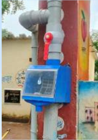
Filter unit for removal of dirt that comes with rainwater
