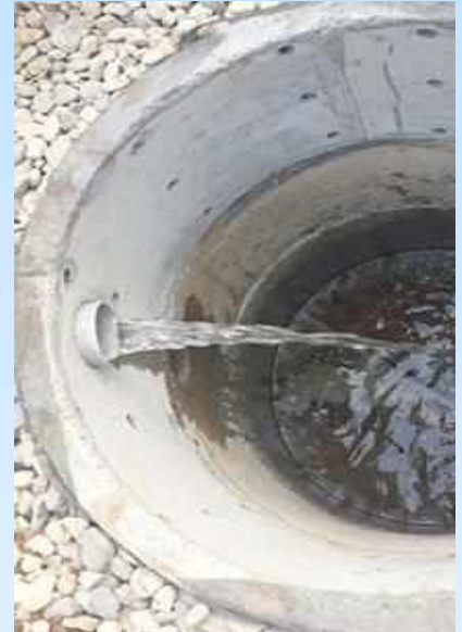
A tank or groundwater recharge structure for storing water
