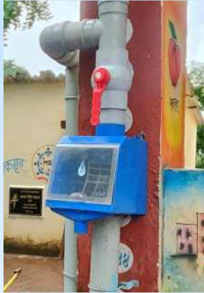
Filter unit to remove dirt carried away by rainwater
