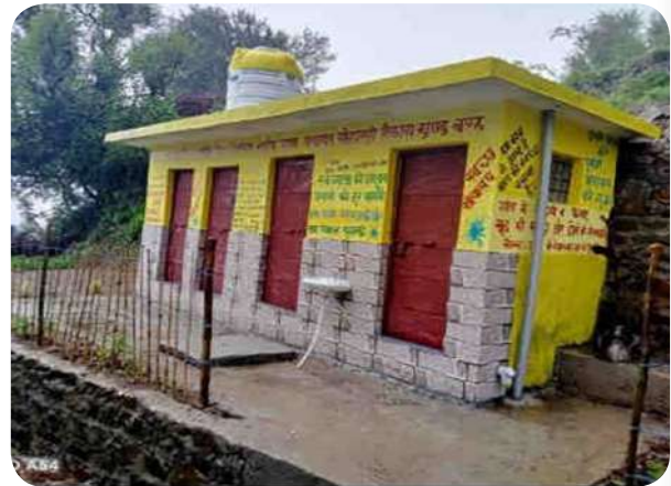
One of the toilets in the GP
