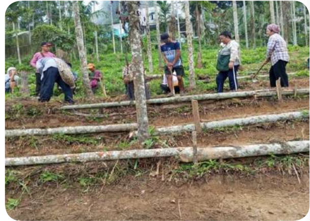
Construction of check dams
