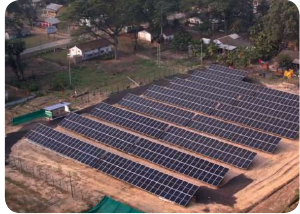
Solar pumps installation through PM-KUSUM Yojana
