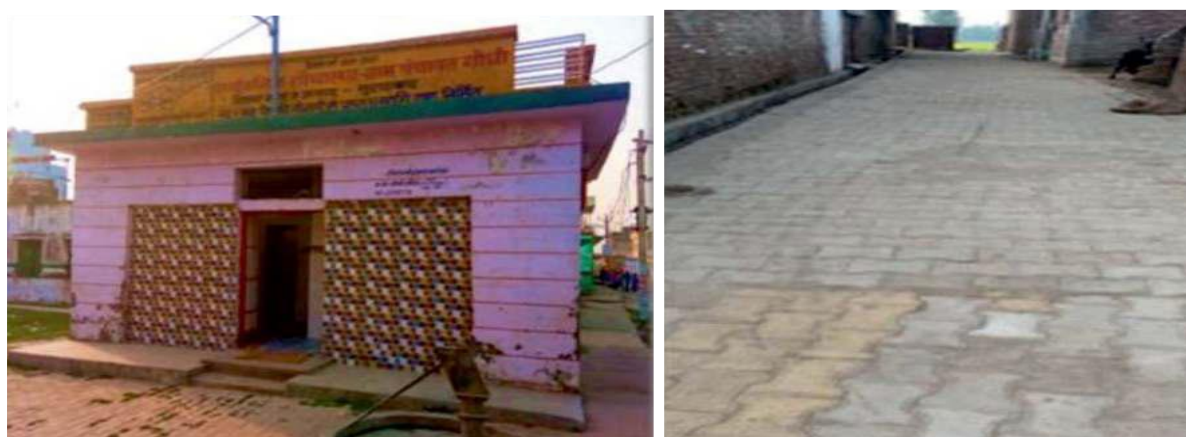
Figure 47: picture from left to right (a) Community Sanitary Complexes (CSC) (b) Construction of Road
