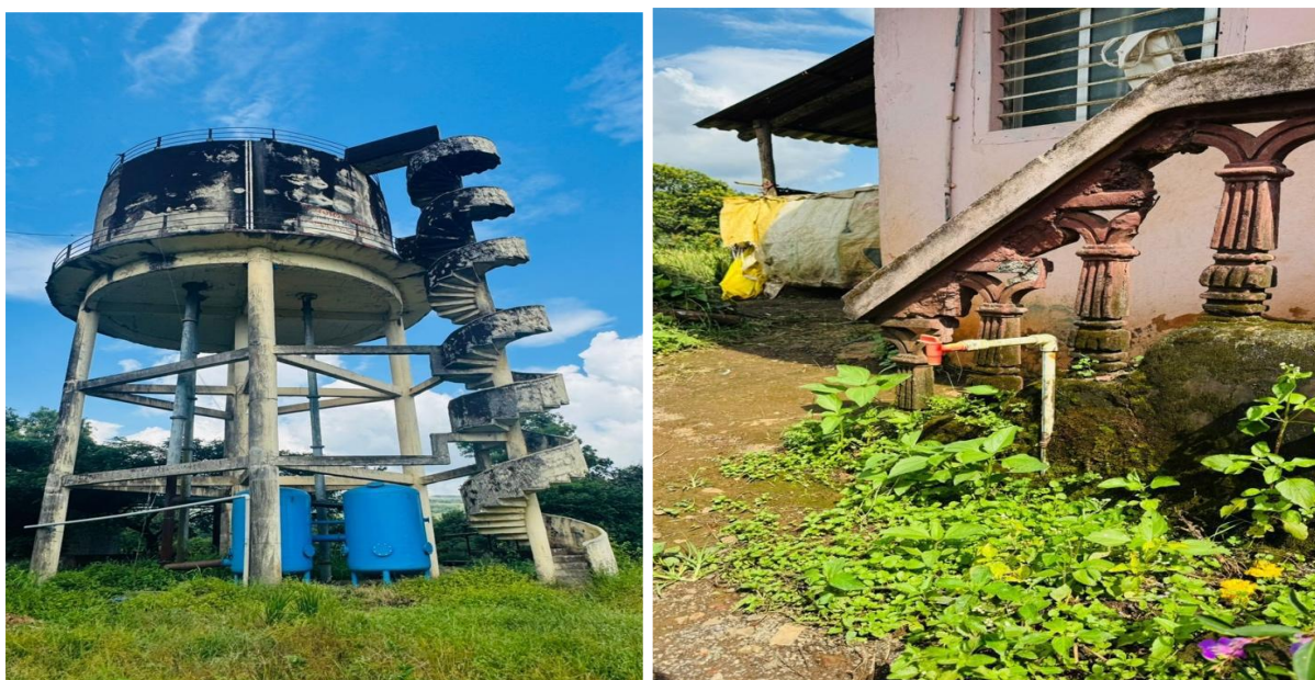
Figure 44: Picture from left to right (a) Overhead Tank at Gram Panchayat (b) Pipeline Water Supply to Households
