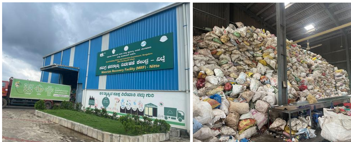
Figure 40: (a) Material Recovery Facility, Nitte (b) Waste Storage Facility, Nitte
