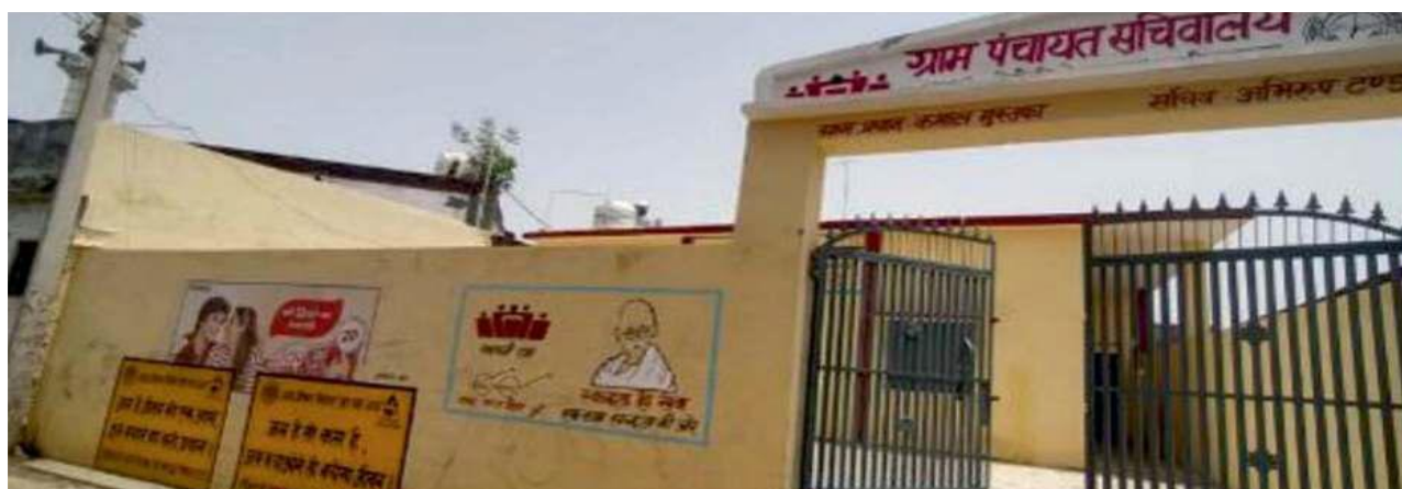
Figure 46: Construction of Panchayat Bhawan
