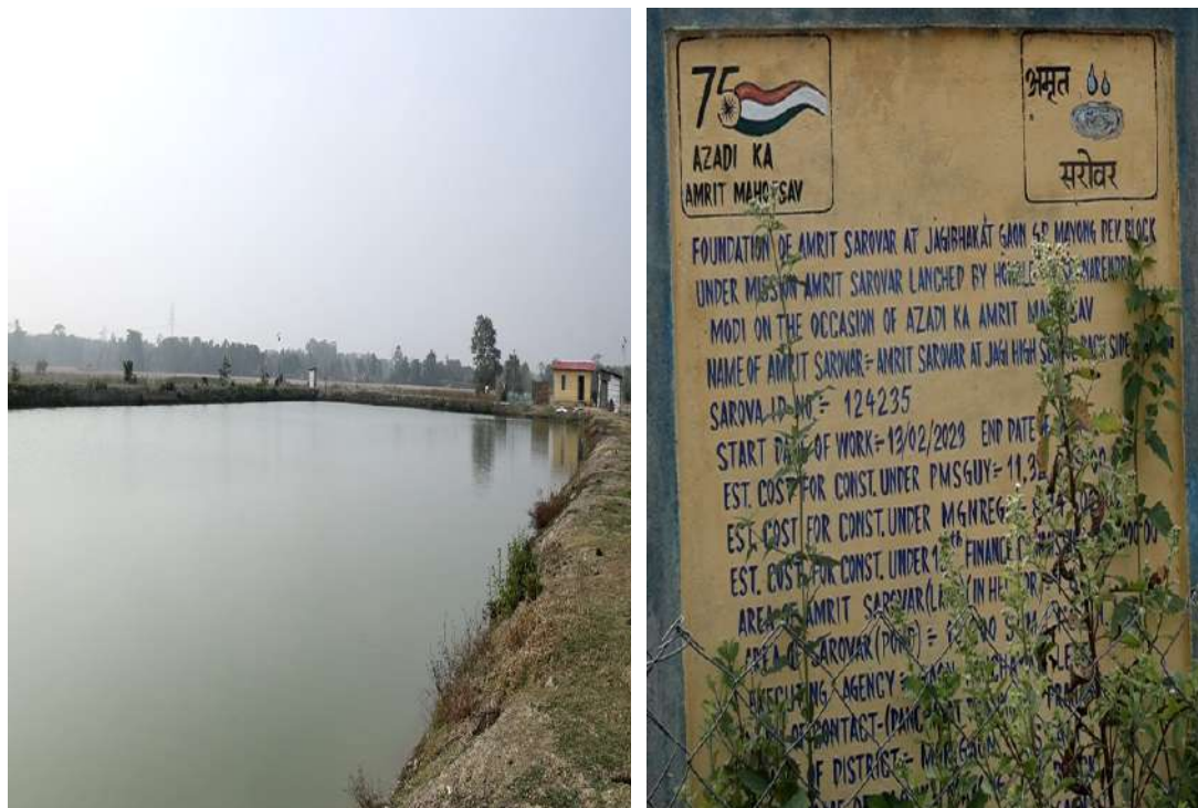
Figure 5.3 : MGNREGA labour employed in Amrit Sarovar construction in Jagibhakat Gaon GP in Assam
