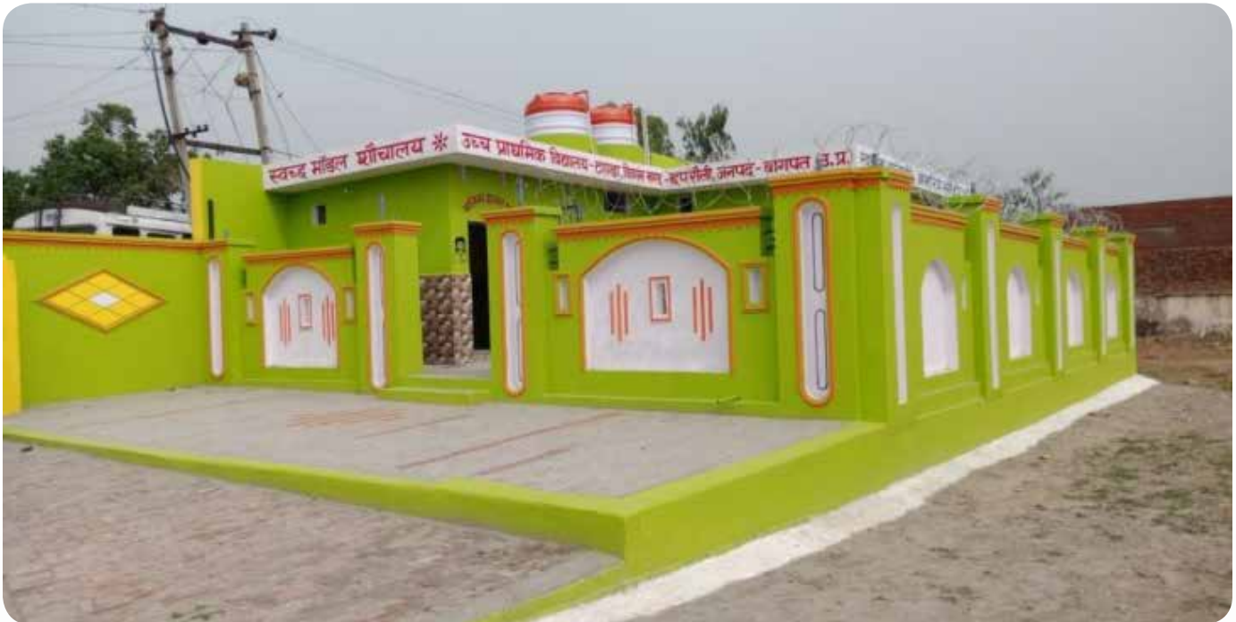
Tanda Gram Panchayat, District-Bagpat, Uttar Pradesh has constructed a model toilet using grant from the central finance commission.
