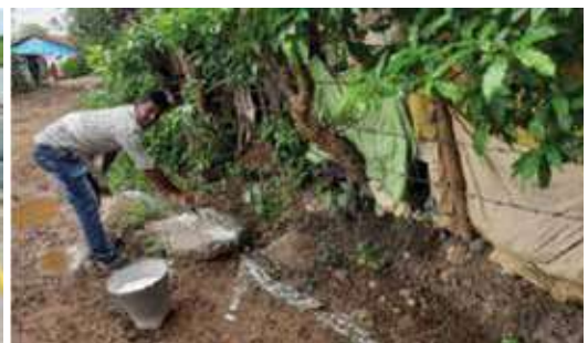
6. Property demarcation using Chuna Powder
