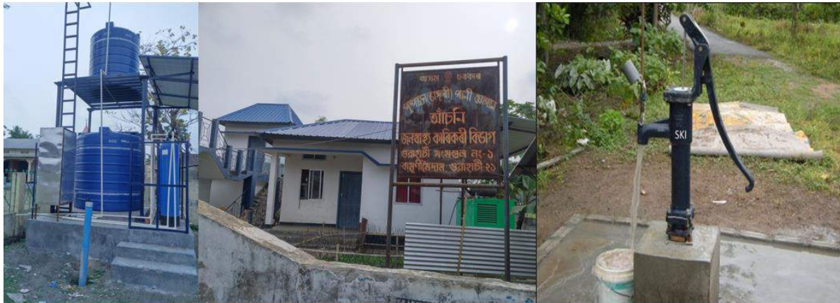
a) Water supply system in school under construction
