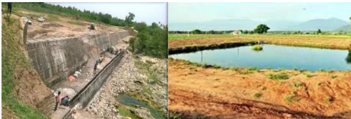
Restoring Tanks / Water bodies for Minor Irrigation
